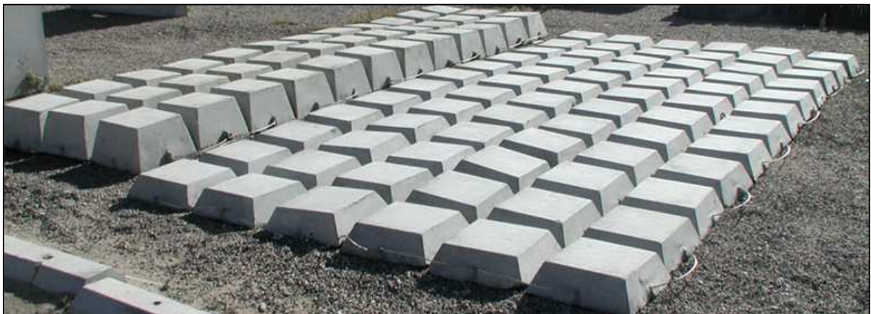
Figure 3. Wet-cast ACB SPS
