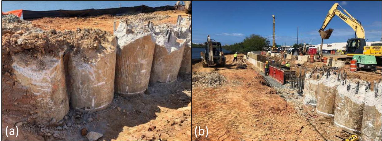
Figure 2. Drilled shaft tangent walls
