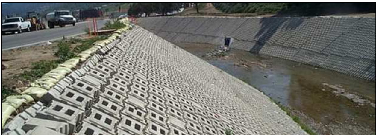
Figure 4. Dry-cast ACB SPS
