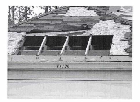
Figure 3.18 – Loss of roof panel picture from hurricane Katrina.
