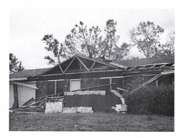
Figure 2.2 – Loss of a porch over-hang due to lack of support post anchorage
