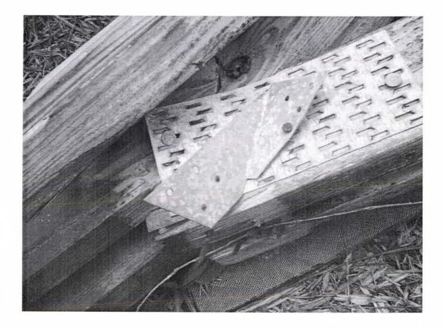
*Figure 2.5 – Photo of missing fasteners in a hurricane clip. The roof lifted off after several hours of uplift pressures.*
