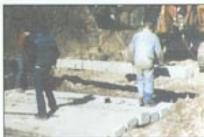
Concrete planks, fastened together and stretched across the streambed, provide an improved ford crossings.
