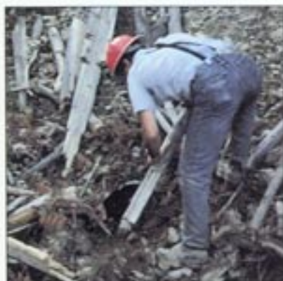
Hand, shovel, and chainsaw work are usually all that culvert maintenance requires. But don't delay! Delay in cleaning a blocked culvert or ditch can result in a damaged road which requires costly reconstruction.
