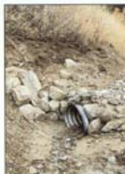
Drop inlets (left photo) installed at the head of a ditch relief culvert slow the flow of water, help settle-out sediment, and protect the culvert from plugging. Rock armored inlets (right photo) prevent water from eroding and undercutting the culvert and flowing under the road.
