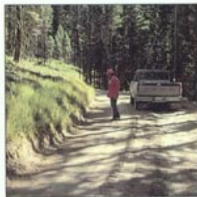
Grader damage to inside ditch toe slopes exposes an easily erodible surface and is a source of sediment. Slow, controlled grading is often the solution, and it can also avoid damage to ditches, culverts, and cutbanks.
