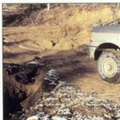
Before grading, it may be necessary to loosen hardened or deep rutted road surfaces. Ripper shanks on a road grader are effective. Road repairs should occur before the wet season. Special attention is needed on steep slopes or curves where greater road surface wear occurs.
