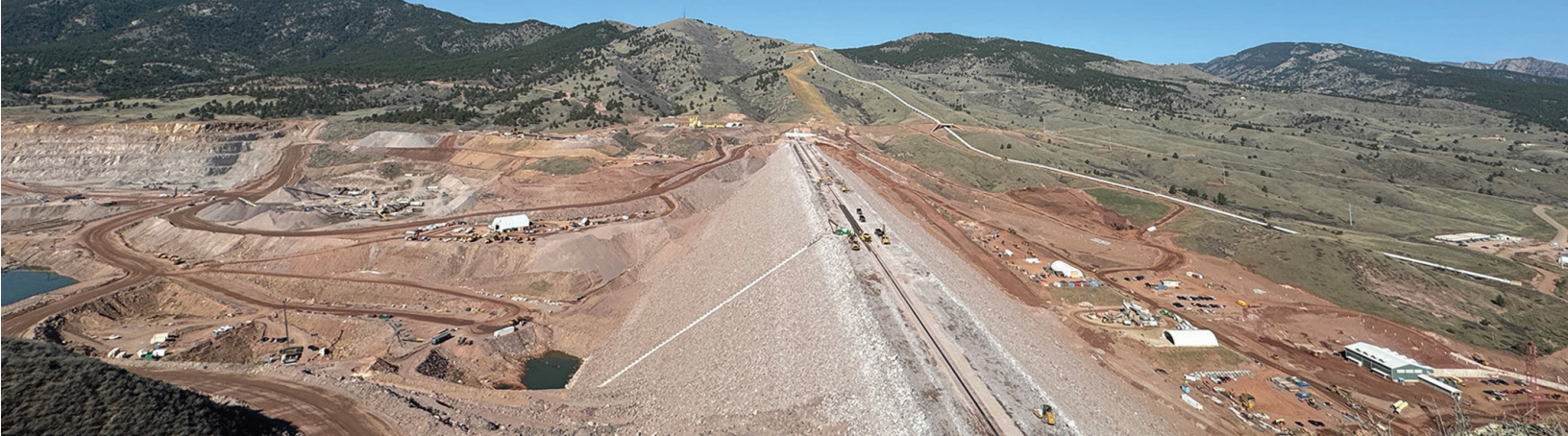
Photograph of Chimney Hollow Dam construction courtesy of Northern Water.
