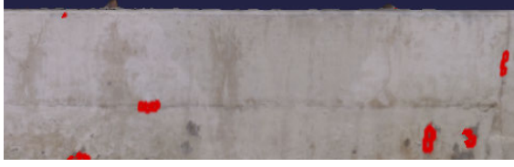
(a) Detected Damage of the Side of the Bridge Using the Texture Technique of Defect Mapping
