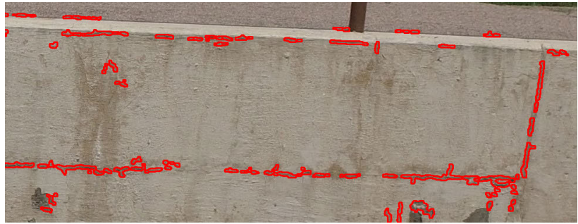
(e) Highlighted Cracked Section
