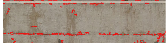
(b) Detected Damage of the Side of the Bridge Using the Original Image in the Defect Detection Algorithm
