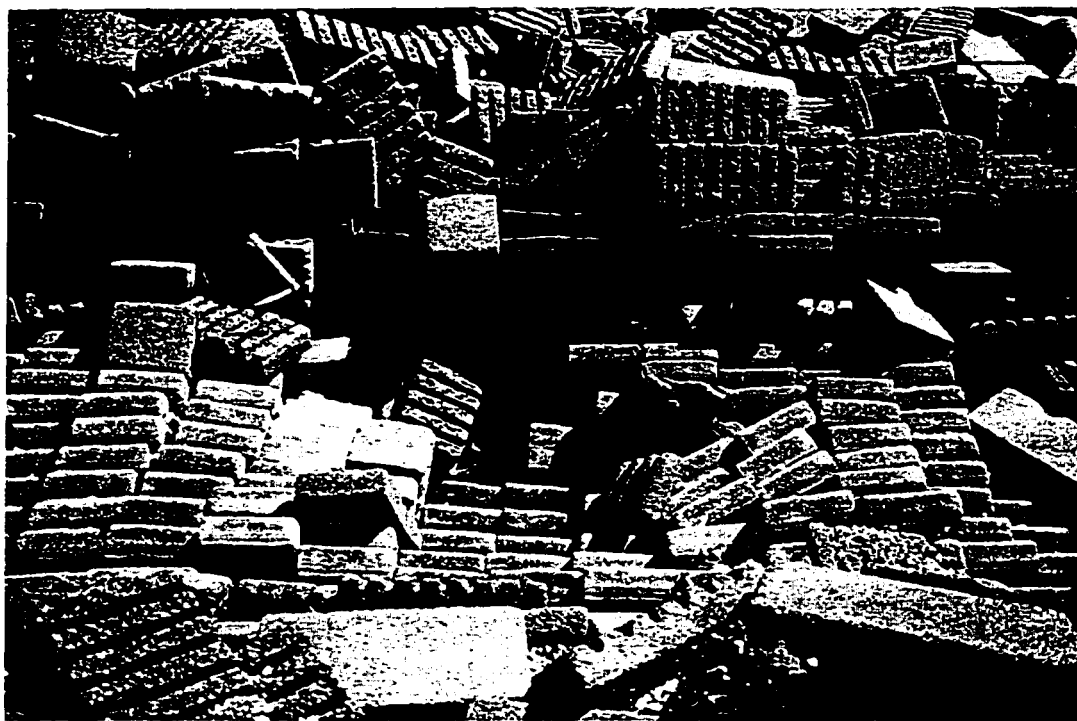
Figure 5.18. Photograph of the scour hole after test conducted at 1.98 \text{ m}^3/\text{s} (70 cfs).
