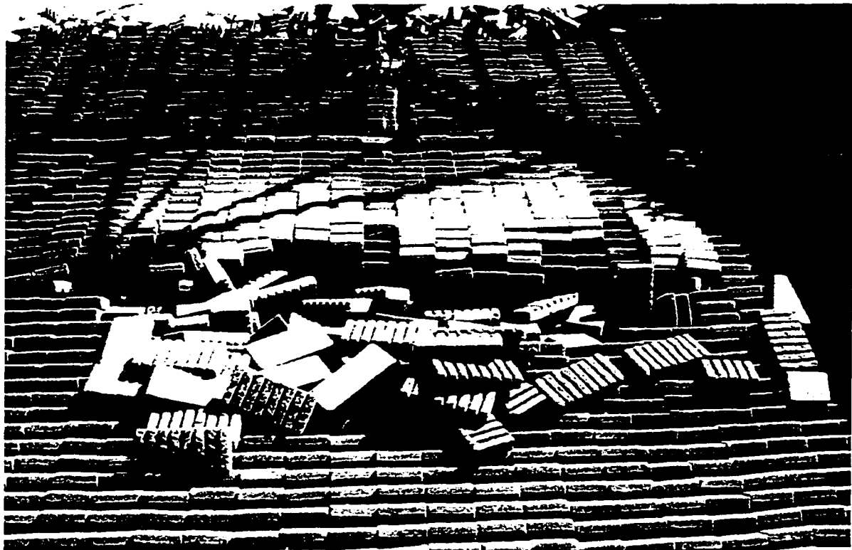
Figure 5.12. Mat after failure at 1.13 m 3 /s (40 cfs).
