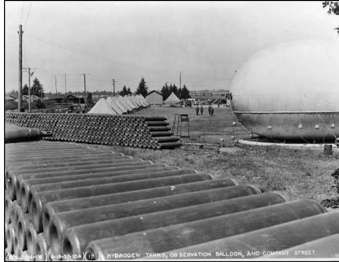
Figure 30: Airship Hydrogen Refilling Tanks [49]
