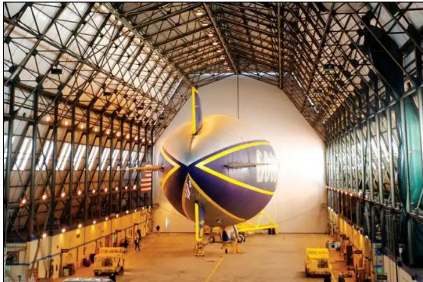
Figure 118: Interior of Goodyear Blimp Maintenance Hangar [156]
