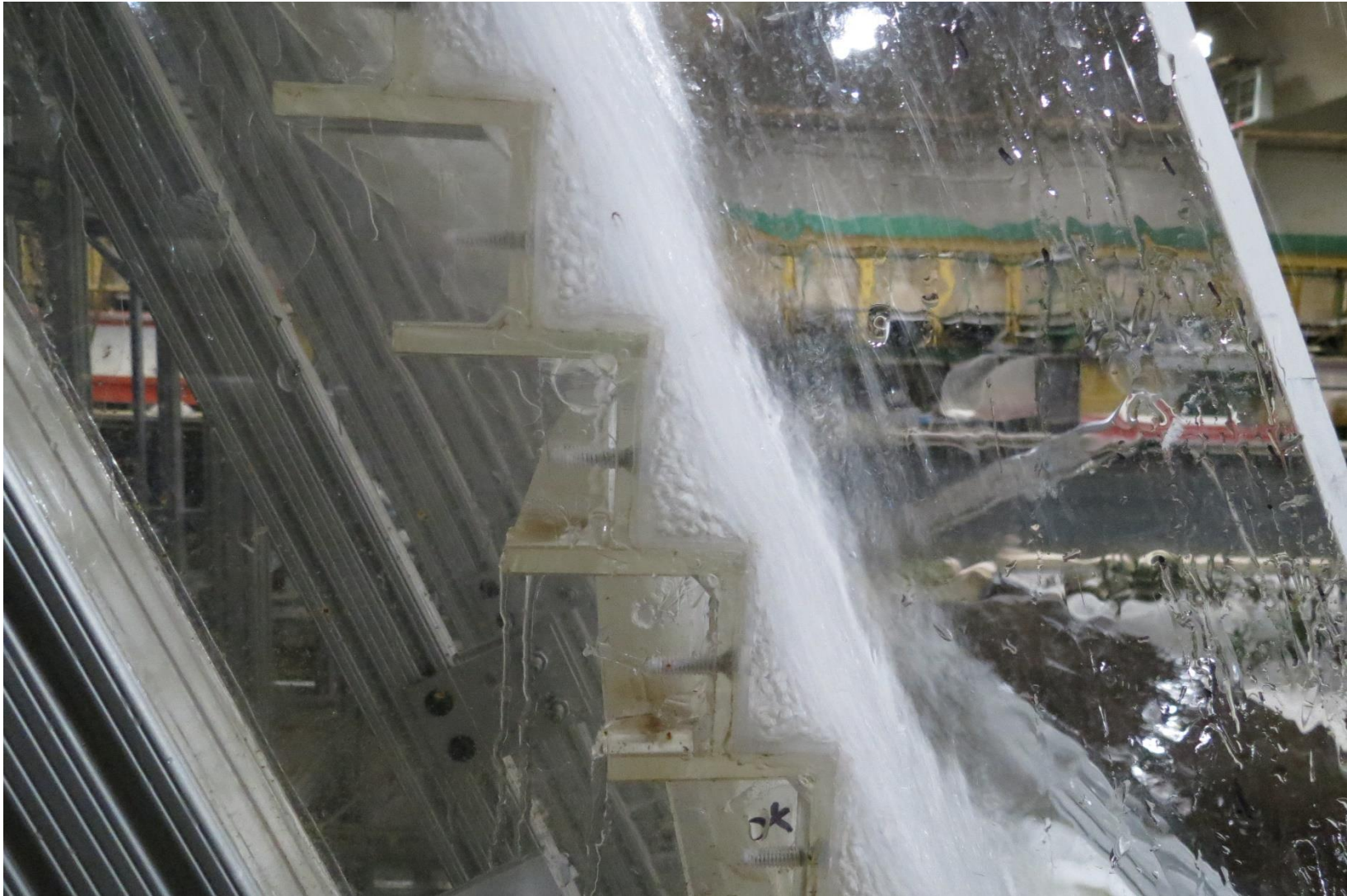
Figure A.8. A photograph of the spillway chute conveying a water discharge of Q = 0.028 \text{ m}^3/\text{s} .
