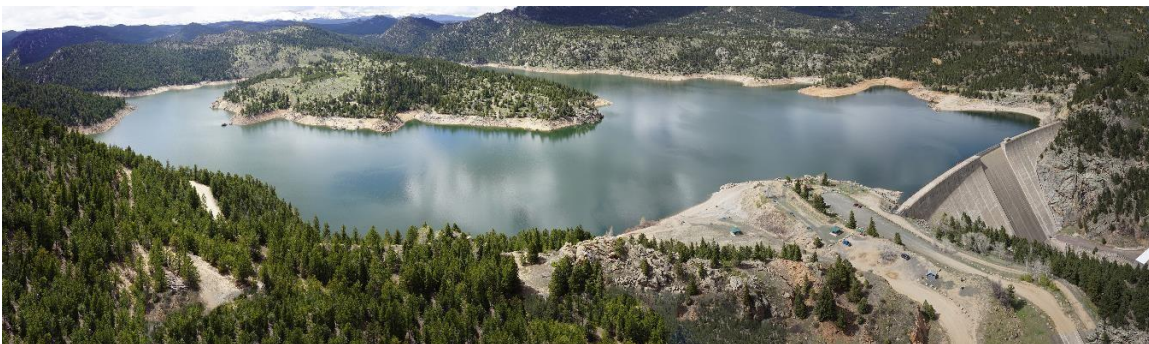
Figure 1.1. A panoramic view of Gross Reservoir and Dam.
