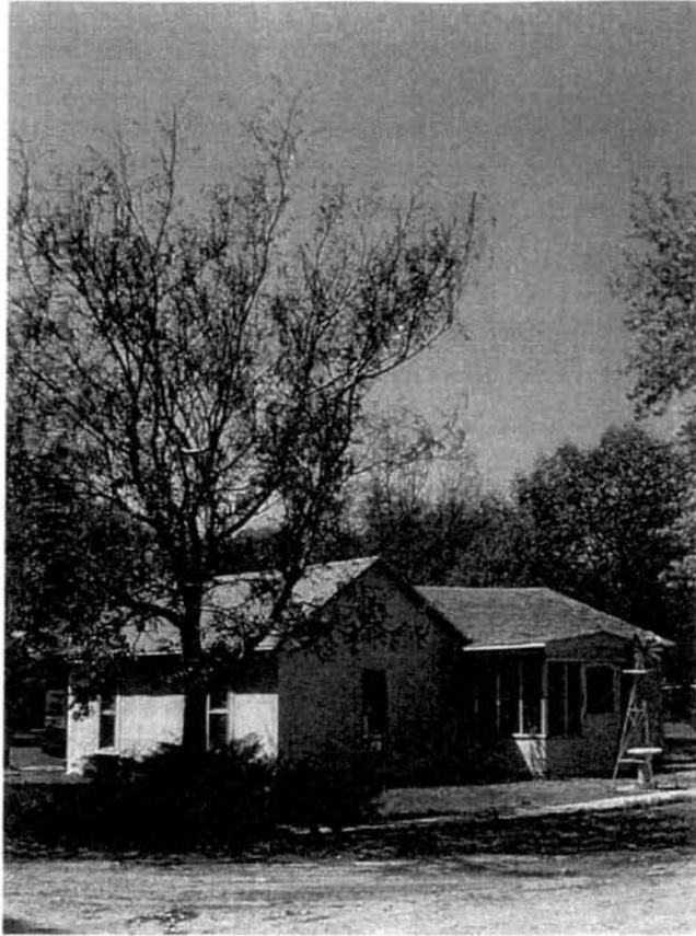
Figure 4.6: Damaged tree in Merino. Note leaves spread across both the ground and the roof of the house.
