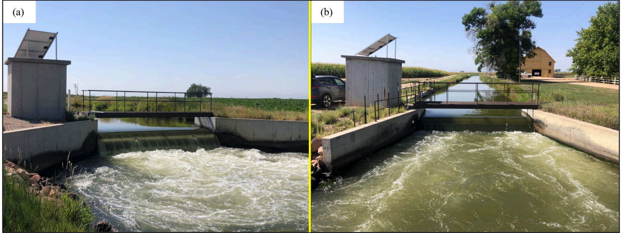
Figure 8.6: (a) Free flow at Weir A ( Q = 4905 L/s; h = 539 mm; \theta = 32.7^\circ ) vs. (b) clinging flow at Weir B ( Q = 4425 L/s; h = 439 mm; \theta = 39.4^\circ ) for the PGV2025 study.
