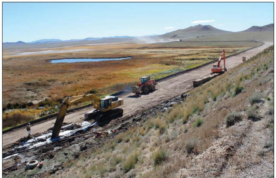
Crews build a sand trench on the downstream side of Antero Dam to filter the normal seepage of the dam and to stabilize the foundation.
