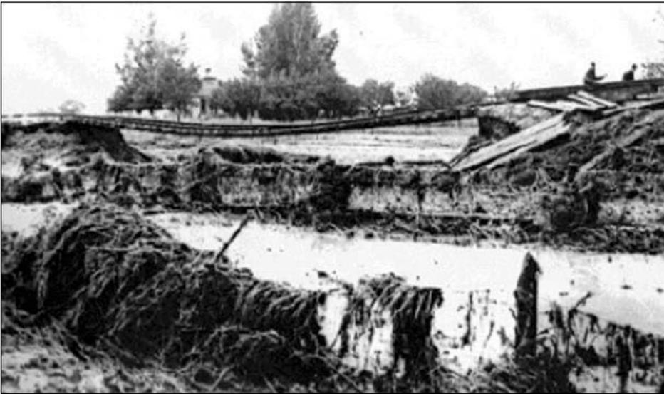
Figure 5. Railroad tracks hanging over the washed-out bed along South Boulder Creek near present-day Highway 93 near Marshall, after the September 1-3, 1938 flood. The gaged peak discharge in the 1938 flood (7,390 cfs) was much higher than that of September 2013, though the latter was influenced by floodwater retention in Gross Reservoir.
