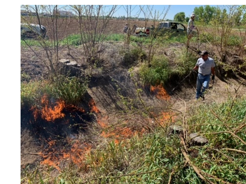
Ditch Burning to clear out the path for water flow
