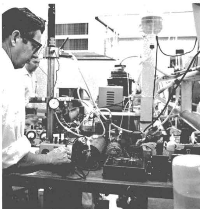
Fig. 1. The Pollak photo-electric condensation nucleus counter Model 1957.
