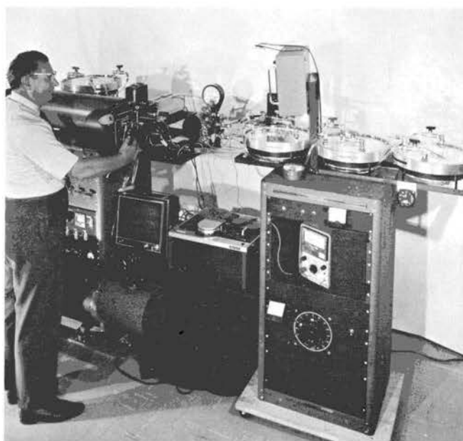
Fig. 2. NRL CCN instrument; thermal diffusion chamber in front of camera (at operator's hand) video camera on opposite side of chamber, video monitor and recorder below; upper left, light source optics; four flat cylinders visible across top are chambers for temperature conditioning of the sample.
