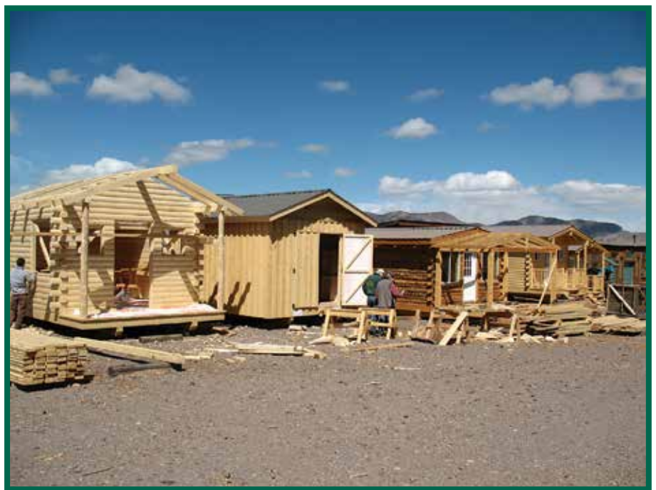
Small-diameter wood can be utilized to create small buildings.
