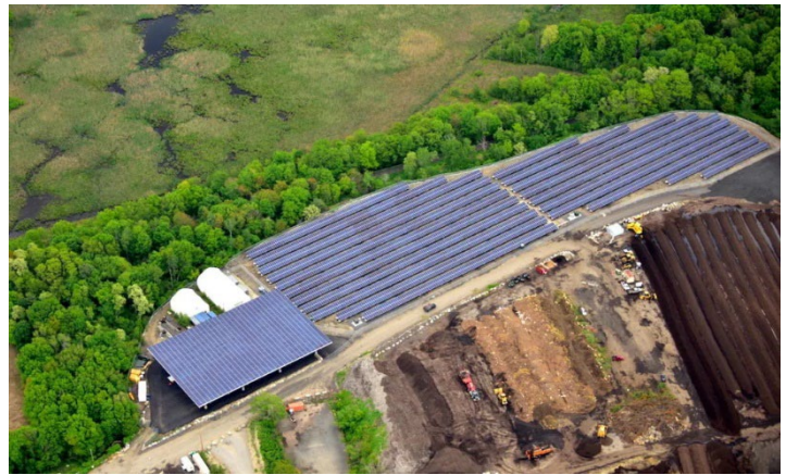
“A Solar Array at a Landfill in Lexington, Massachusetts.”
