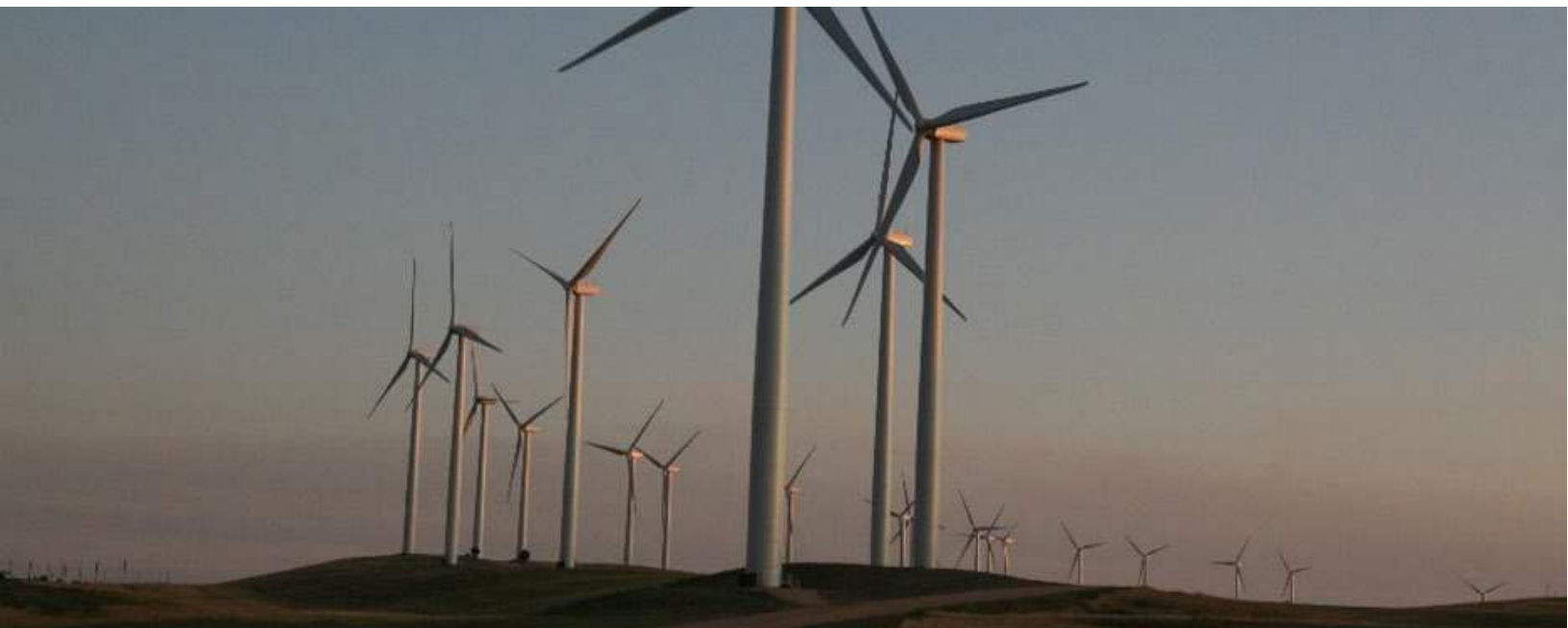
158-unit 237 MW Wind Farm on the Dave Johnston Coal Mine, Wyoming.
