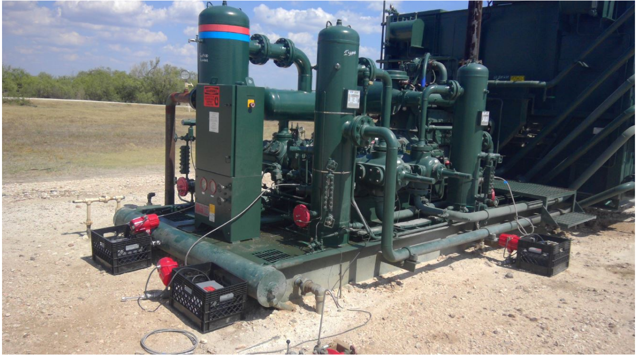
Figure 4.2: Three emission measurement systems installed on exhaust ports to PCs controlling liquid levels on compressor interstage knockout tanks.
