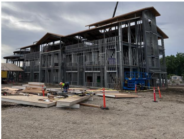
Fig. 2.1. Typical commercial construction that uses steel stud framing. This photo is taken of one of the study sites.
