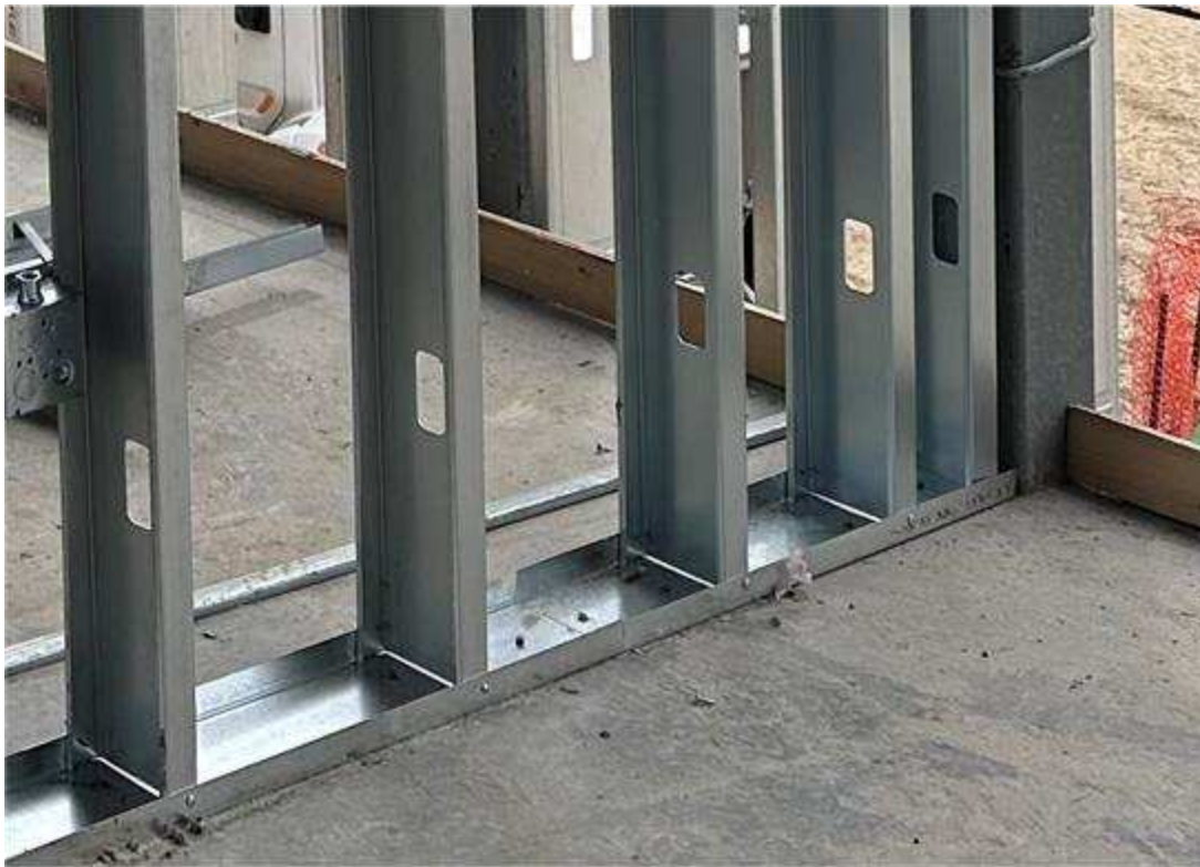
Fig. 1.1. Example of steel stud framing. Vertical studs are attached to the track mounted on the floor.
