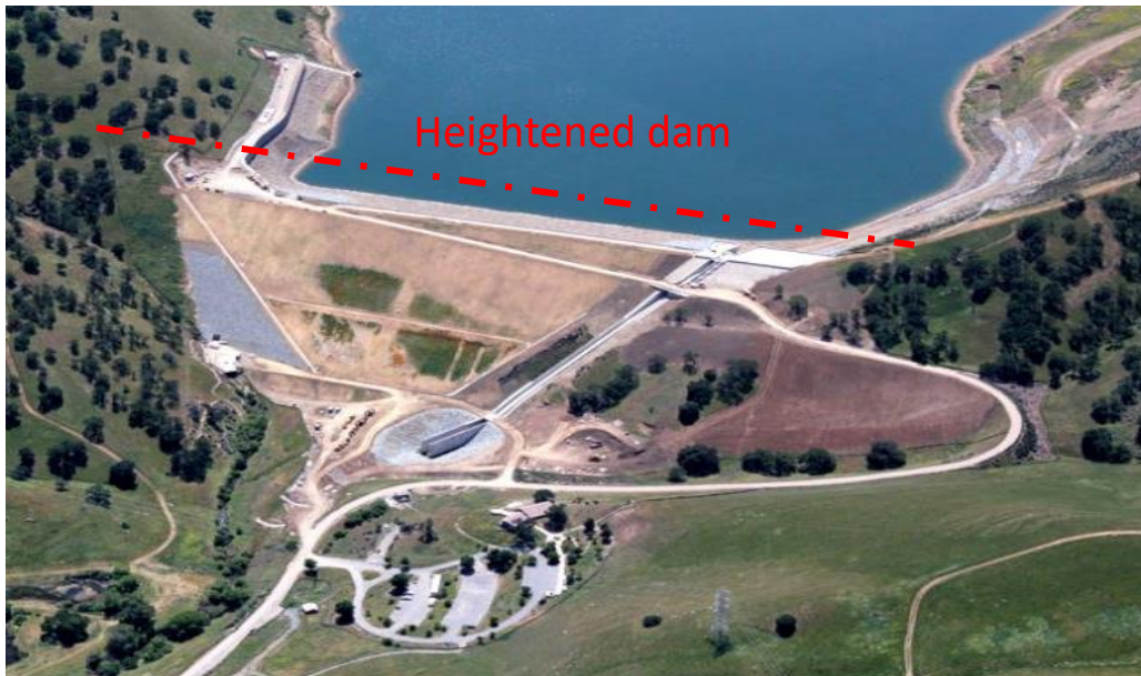
Figure 1-2. Existing dam and proposed heightened dam indicated. (The dam is to be heightened c. 18 m; but the stilling basin is to be retained.)
