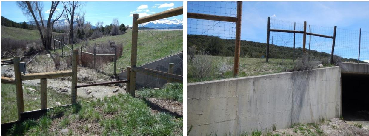
Figure 3. Escape jumps along Dry Creek from the right-of-way above the creek (left) and Alkali Creek from the creek bed (right).
