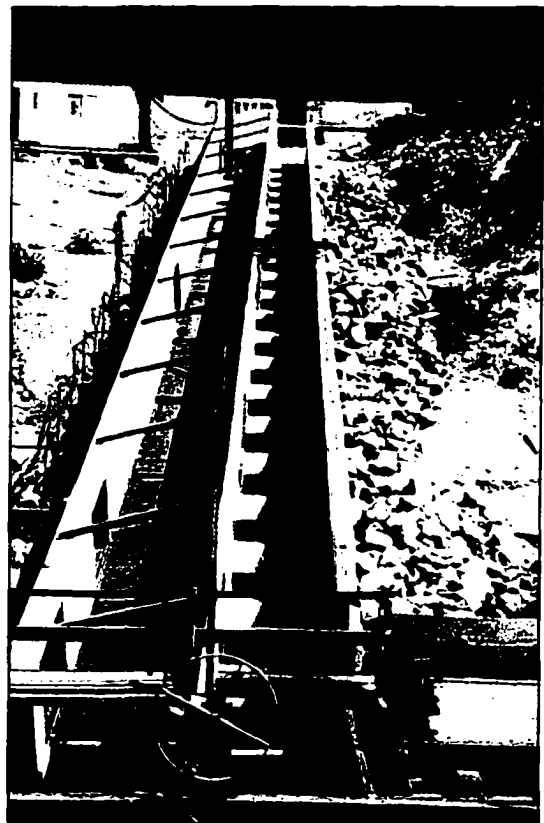
Figure 3.3 – Stepped Spillway, h = 1.0 ft (note: 1.0 ft infills are shown not painted.)
