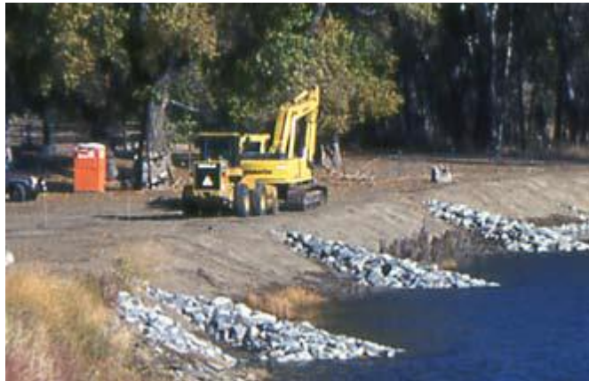
Figure 2. Installation of rock vanes (NRCS 2007)
