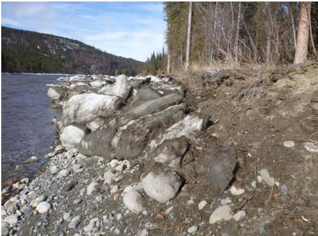
Figure 5-8. Possible remnant shear wall and ice grounding. The shear wall acts to protect the bank toe. Photo taken by HDR Alaska, Inc. on May 10, 2012.
