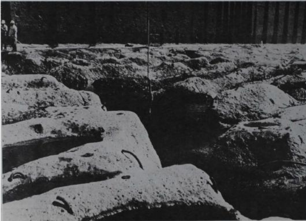
Figure 52. Abrasion-Erosion of Dworshak Dam Stilling Basin Floor (Source: USACE, 1981)
