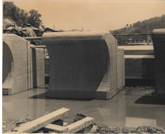
b) Newly Constructed Baffle Block
