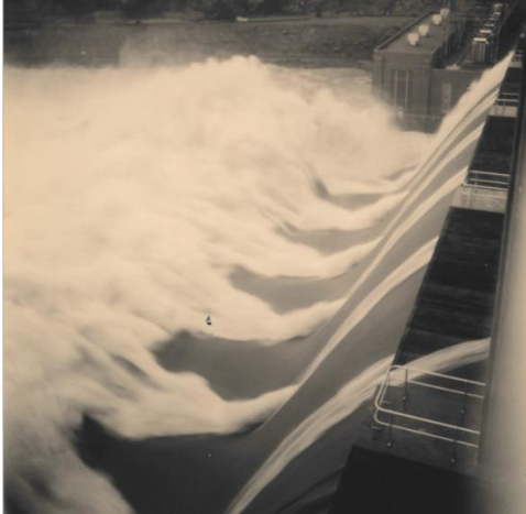
a) Aerial View of Spillway
