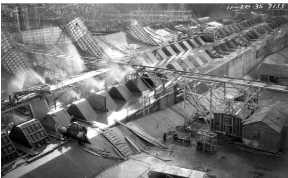
c) Formed/Completed Baffles
