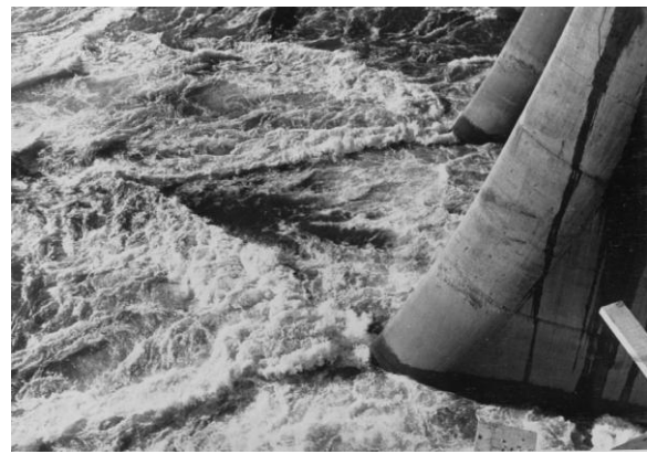
b) Flow conditions on stilling basin
