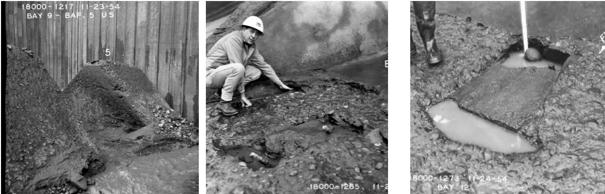
a) Downstream View of Baffle Pier Prior to Cleanup
