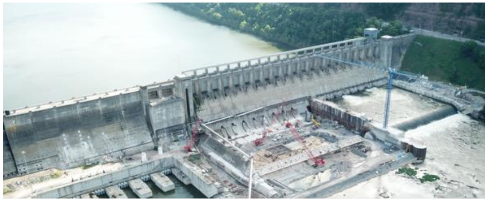
Figure 9. Bluestone Dam Stilling Basin Modification Construction (Photo by Author)
