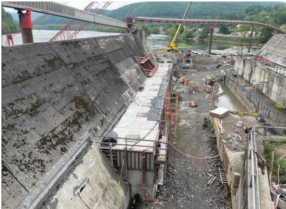
a) Right deflector wall
