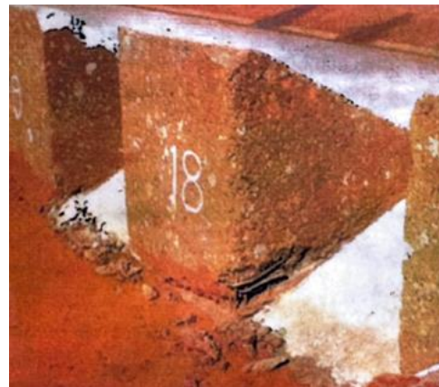
b) Dentated End sill
