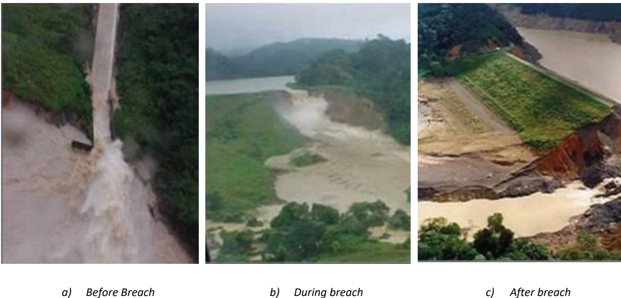
Figure 11. El Guapo Dam Failure (Source: Suarez and Suarez, 2016)
