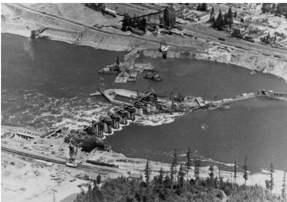
a) Aerial view of River Diversion into South Half of Spillway
