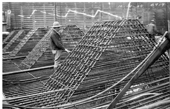
d) Baffle Reinforcement
