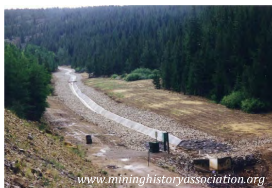
Superfund clean-up in California Gulch involved capturing run-off and channeling it away from mine waste piles.
