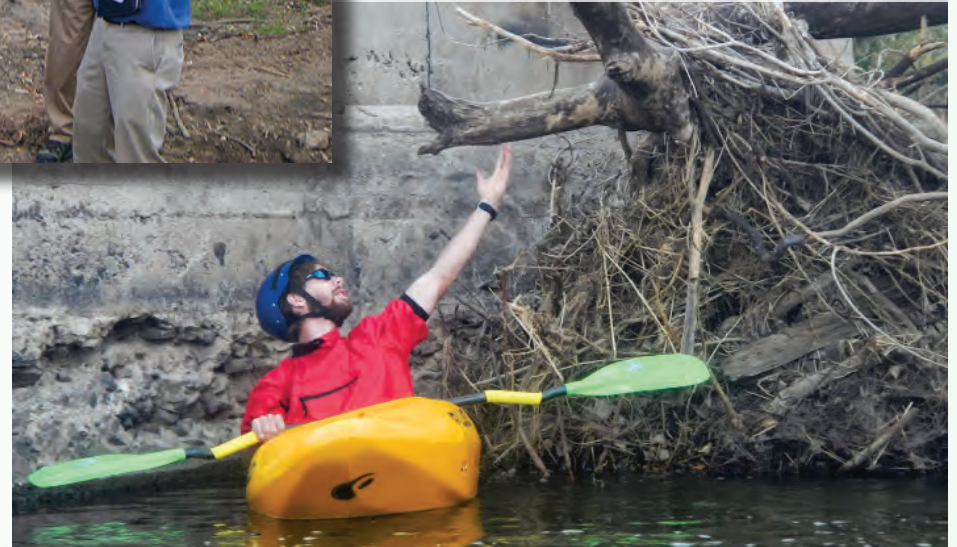
Wood piled against a train bridge pier on the Poudre River near Greeley after the Fall 2013 flooding. Photo by Natalie Anderson
