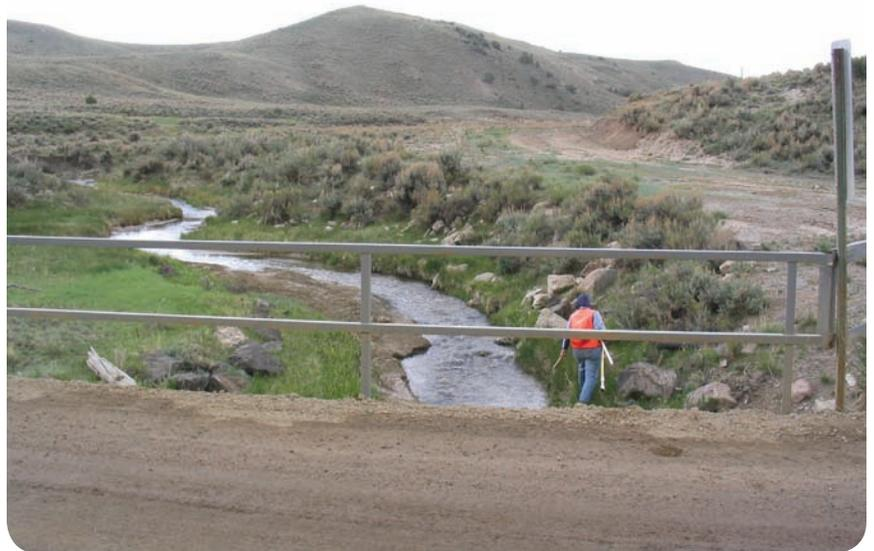
*Stream crossing under a non-paved road treated with  $MgCl_2$  for dust suppression.*
