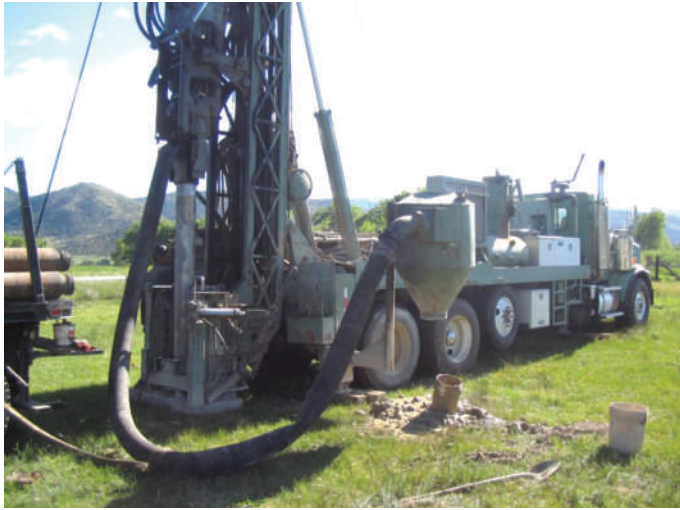
Figure 2.8. The 35-ton dual-wall percussion-hammer drill rig.
