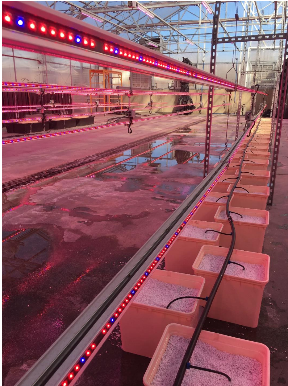
Figure 2. Interlighting system with two sets of light bars (13:3 red:blue diodes per 23cm) and perlite-filled Bato buckets prepared for hydroponic production of greenhouse tomatoes.
