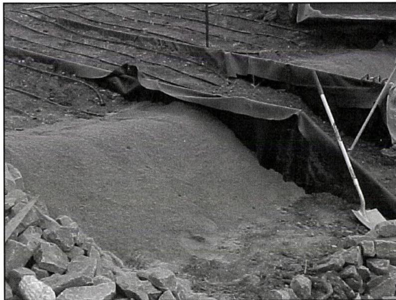
Fig. 3.11. Coarse sand layer on bank slope in Cell A.
