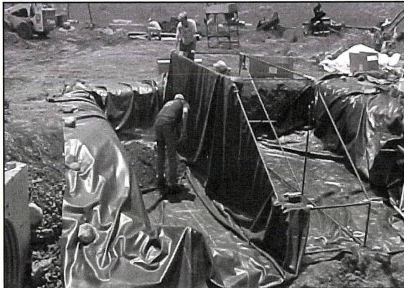
Fig. 3.6. Placement of impermeable liner in research cell.
