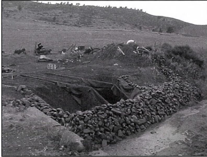
Fig. 3.8. Longitudinal peaked stone toe protection with tieback.
