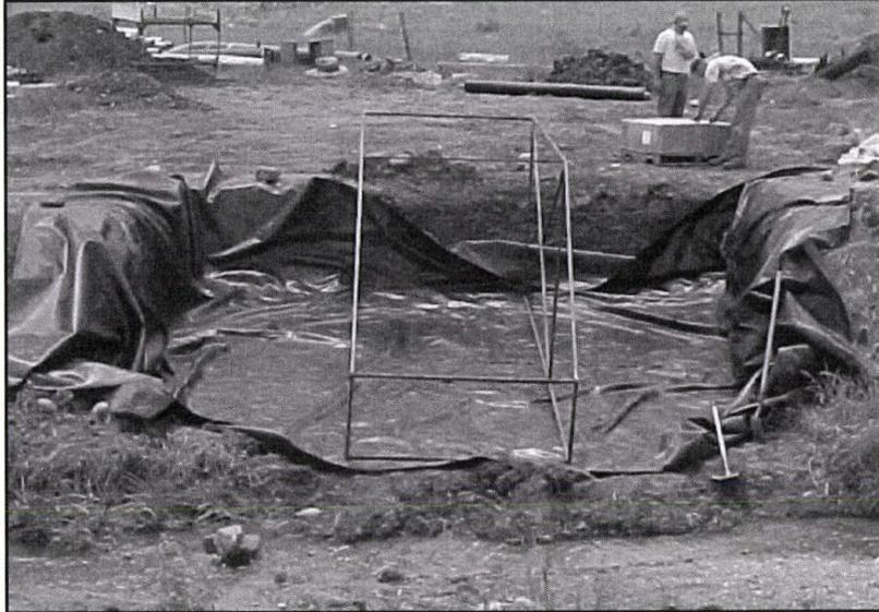
Fig. 3.5. Placement of filter fabric and steel frames.
