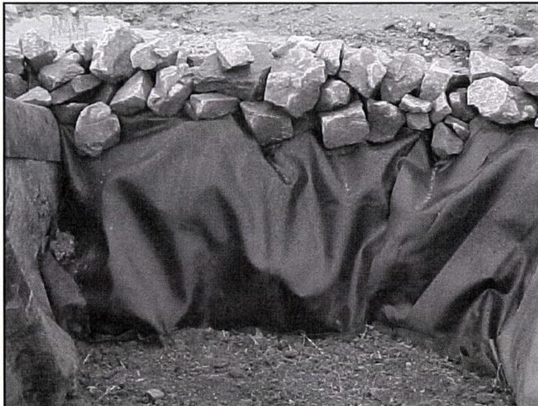
Fig. 3.9. Placement of filter fabric along slope of stone toe.
