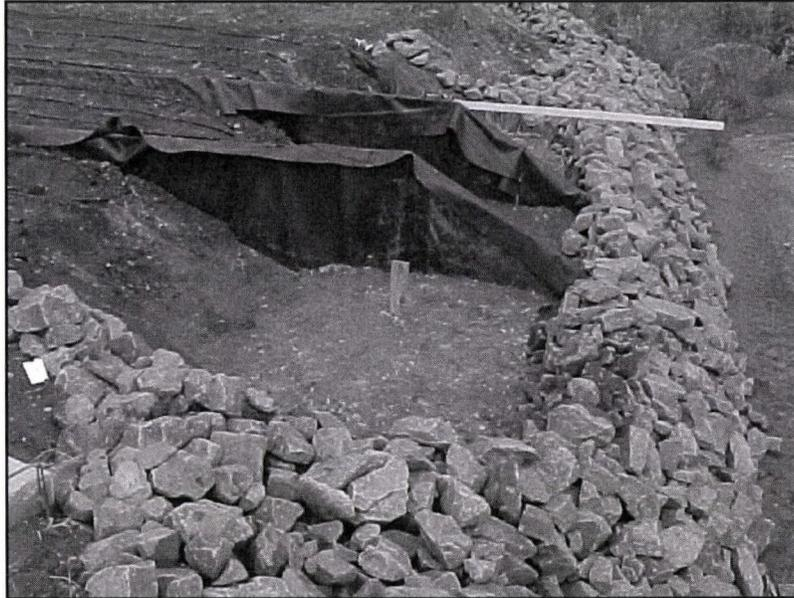
Fig. 3.10. Reactive stream stabilization (RS2) structure in Cell A.
