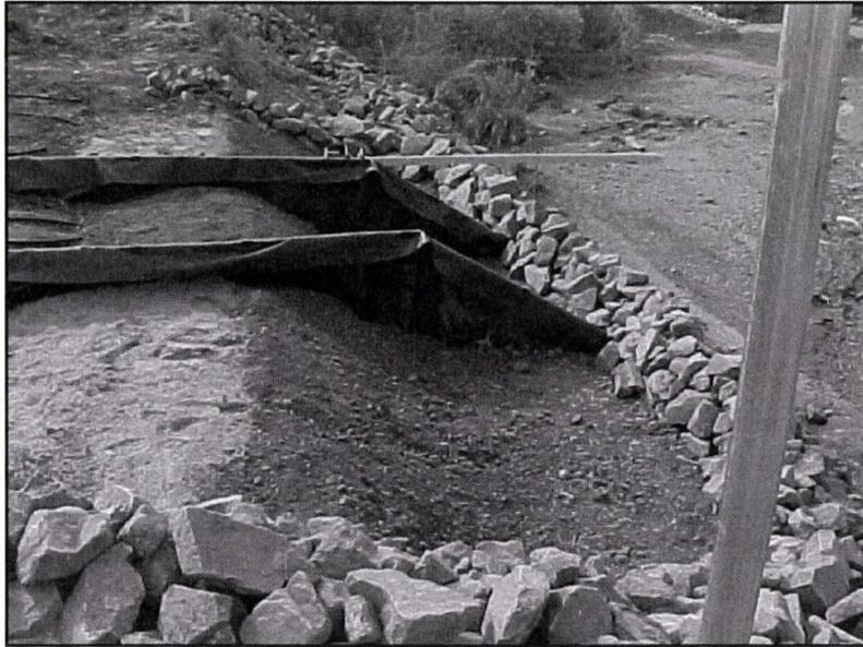
Fig. 3.12. Native soil covering sand layer and reactive barrier.
