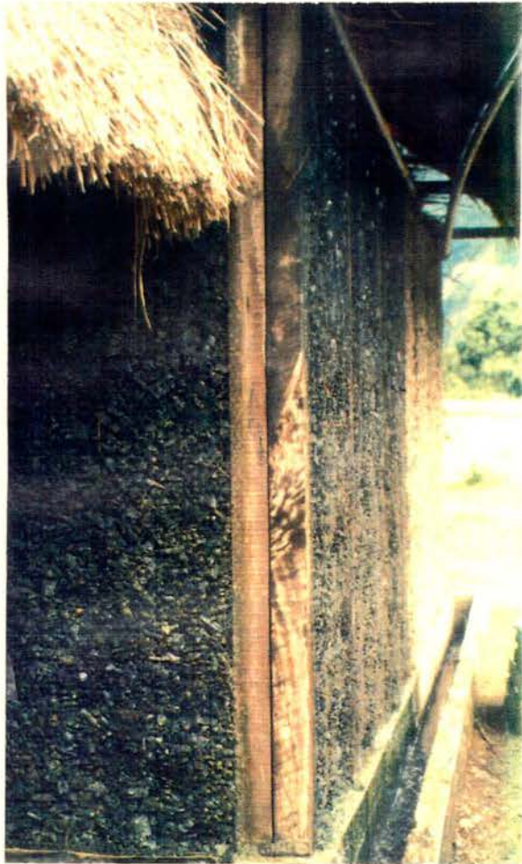
Figure 3. Left:Pipe with holes (left one) allows water to trickle down the charcoal wall. Right:Farmer's Storage at San Ramon.
