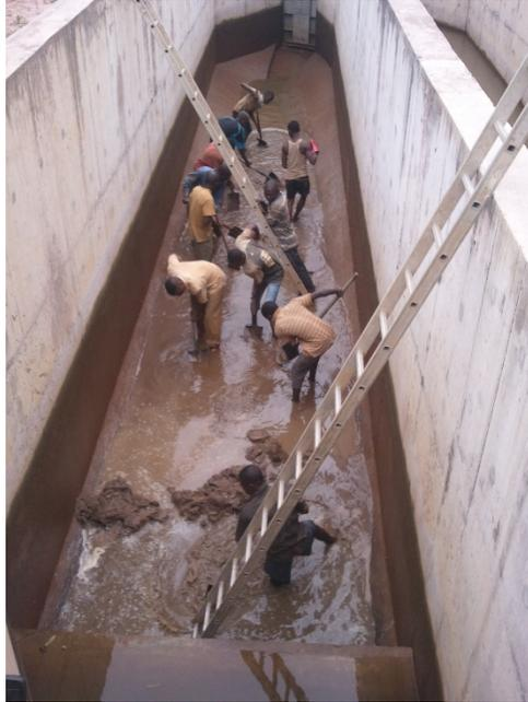
**Figure 1.7 – Cleaning operations of diversion canal of the Lukaya water plant (Picture: Regideso, 2013)**
