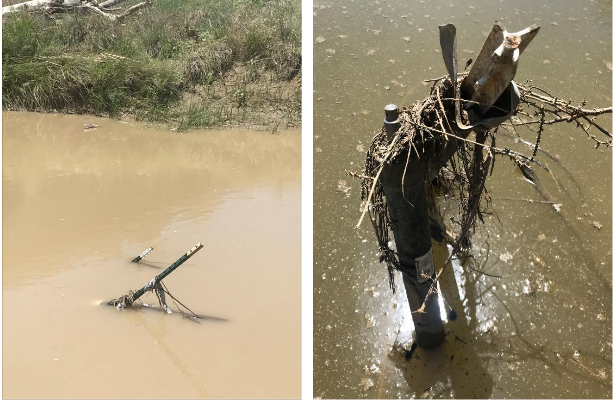
Figure 14. Images of the challenges faced throughout this research: large flows knocked out telemetry system and washed away one logger at PURLASCO (left image), and large flows caused irreversible damage and forced reinstallation at PURNINCO (right image).
