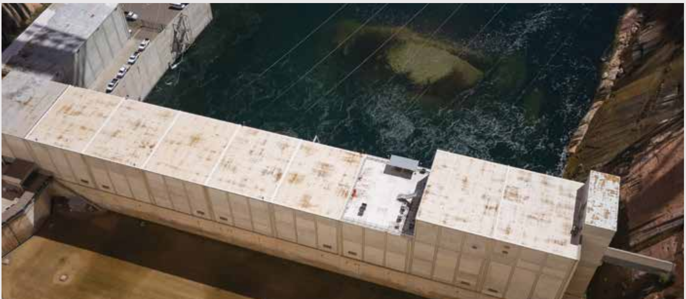
The hydroelectric power facility at Glen Canyon dam has a total capacity of 1,320 megawatts and produces about five billion kilowatt-hours of hydroelectric power annually which is used in Wyoming, Utah, Colorado, New Mexico, Arizona, Nevada, and Nebraska. Photo ©iStock.com.
