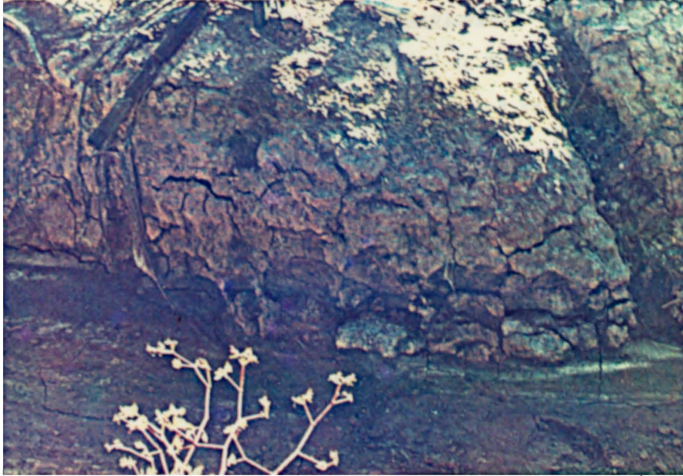
Photograph 2. Mechanical failures of ephemeral gully banks, limiting gully depth. (WES Field Study Site #1, near Vicksburg, Miss.)
