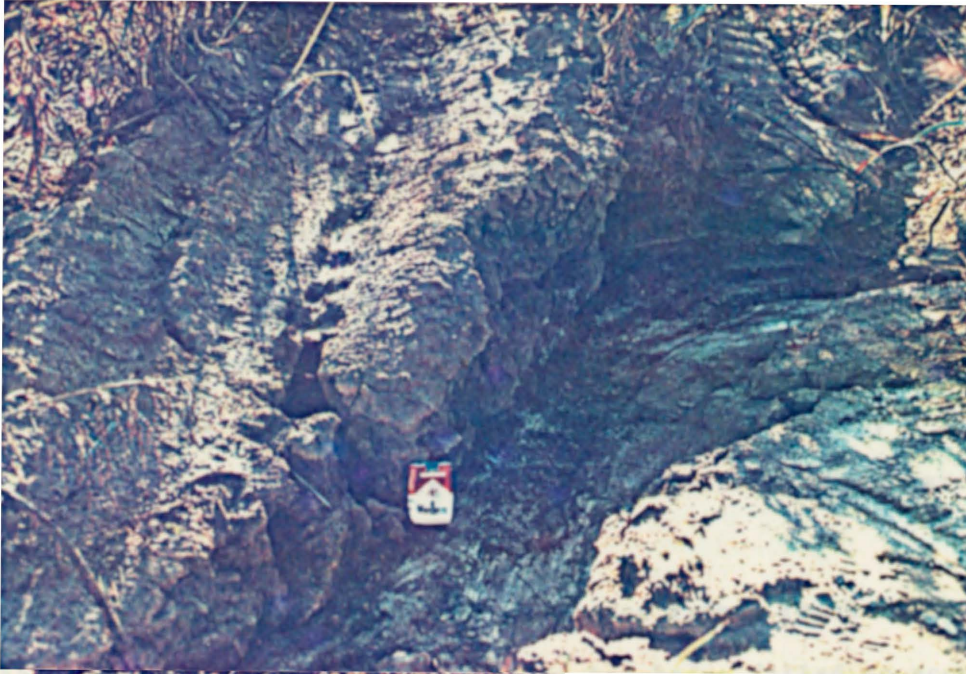
Photograph 4. Degradation of furrow resulting from ephemeral gully degradation. Headcut in furrow to left of center gully has overfall of about 6 inches. (WES Site #1, near Vicksburg, Miss.)
