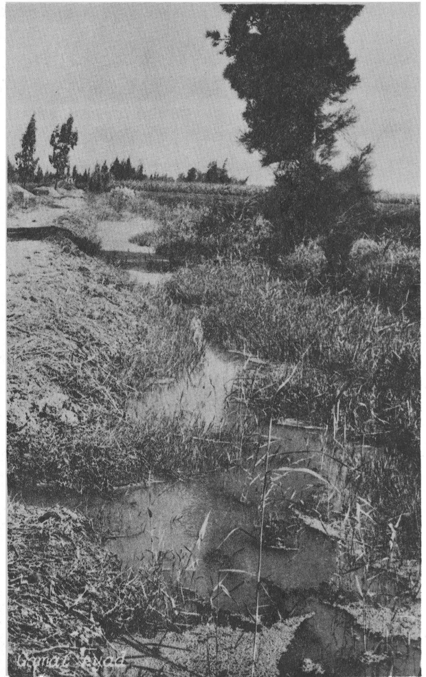
Drains become ineffective because of weed growth. Organizing effective community action to clean drains and canals is an important objective of EWUP.
