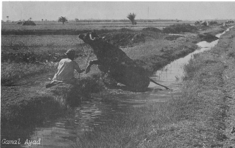
The water-loving buffalo is especially destructive of canal cross sections.
