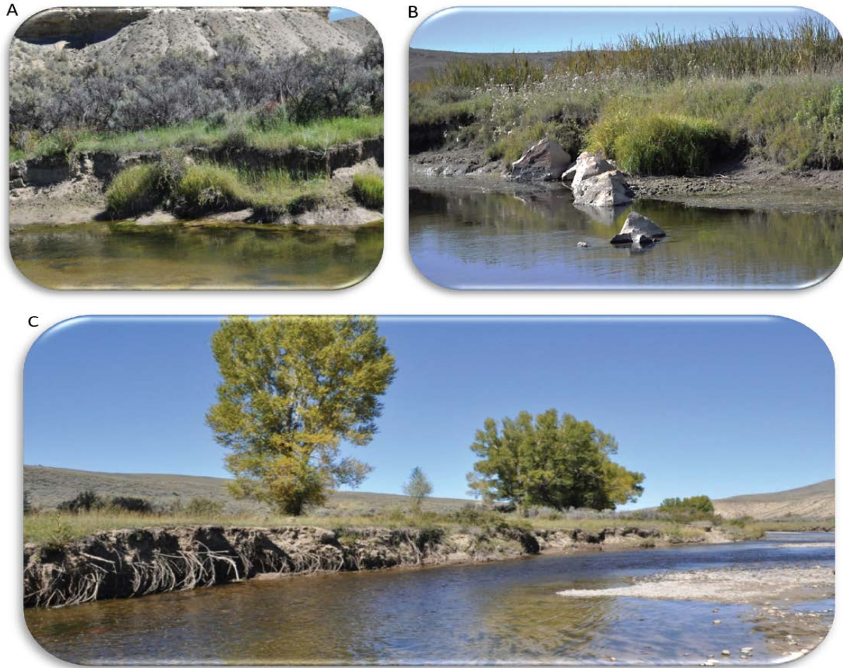
Figure 5. Photographs showing (A) mass wasting or block failure, (B) flanked j-hook, and (C) exposed roots indicative of recent streambank erosion in Muddy Creek below Wolford Mountain Reservoir, September 16-27, 2013.
