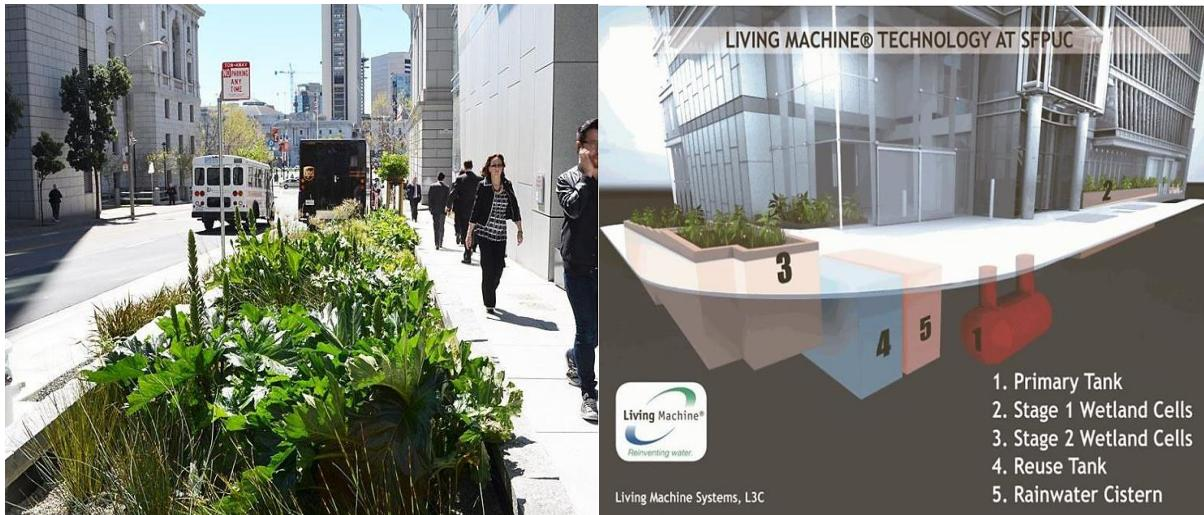
**Figure 2.5 Photograph of Living Machine® Constructed Tidal Wetlands (left), Schematic of Living Machine® Technology (right) (Living Machine, 2012).**
