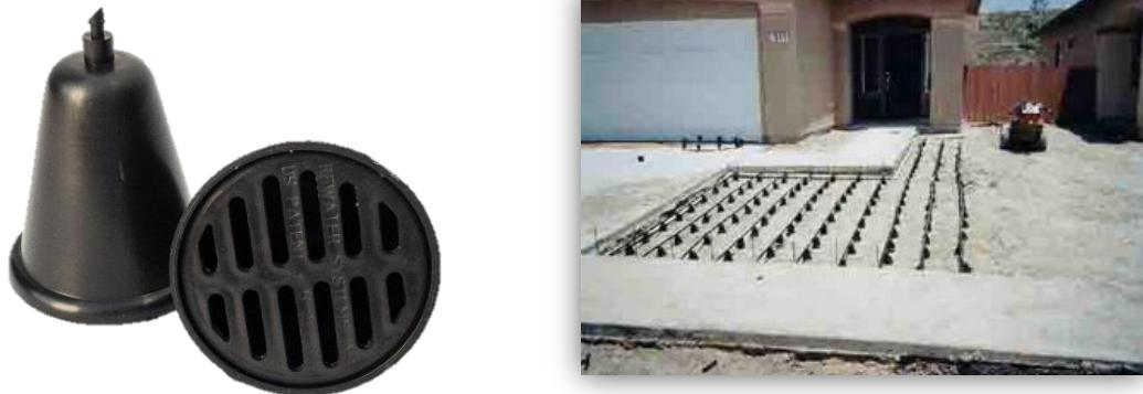
Figure 6: ReWater emitters (left) and emitters being installed under turf lawn for subsurface irrigation (Rewater®, 2014 [Link](#))
