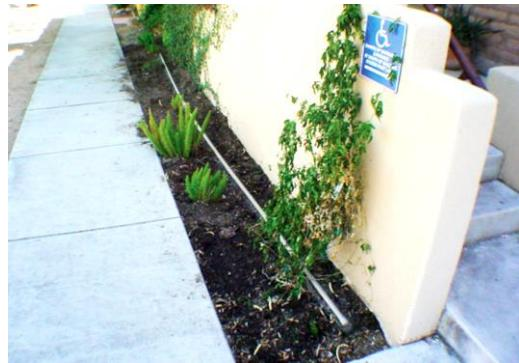
**Figure 2: Drip Irrigation Utilizing Graywater**
