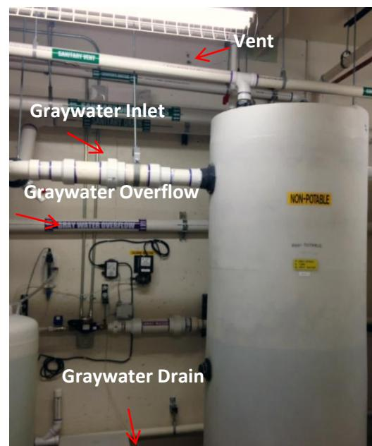
**Figure 5: Graywater Tank and Components**
