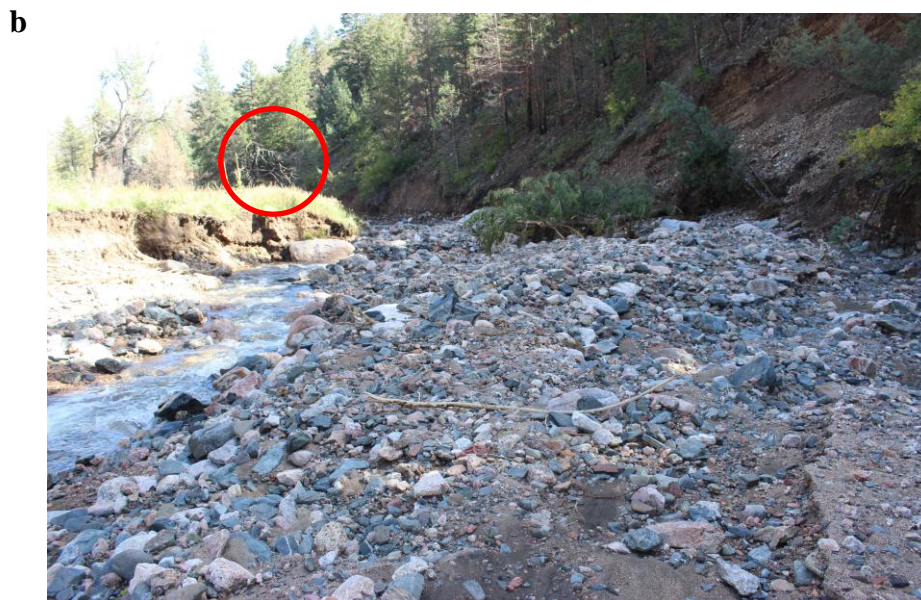
Figure 10. Photos looking downstream at XS4, with (a) being prior to the September 2013 flood, and (b) the same location after the flood. Note the same tree in the upper left of both pictures and the slope failure along the hillslope to the right.
