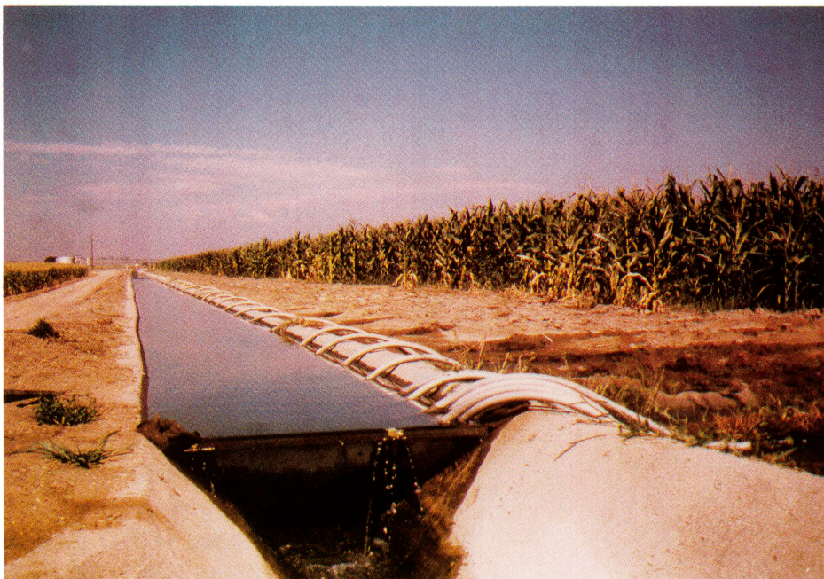
Concrete lined ditches reduce seepage losses.
