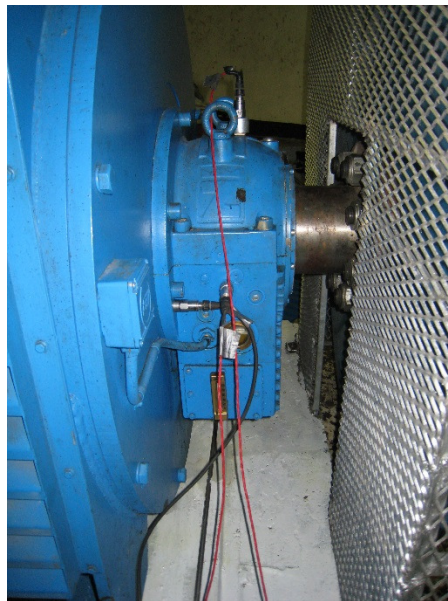
Figure 1. Accelerometers mounted to a bearing housing for vibration measurements.
