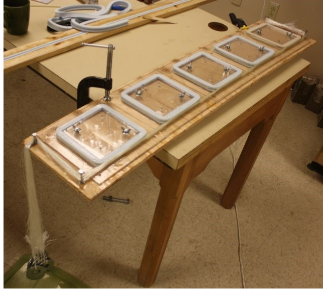
Figure 36: GFRP lay-up of stirrups
