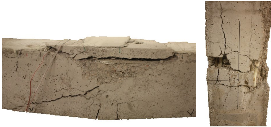
Figure 75: Surface constrictive cracking in Ila-1 (left: side view, right: bottom view)
