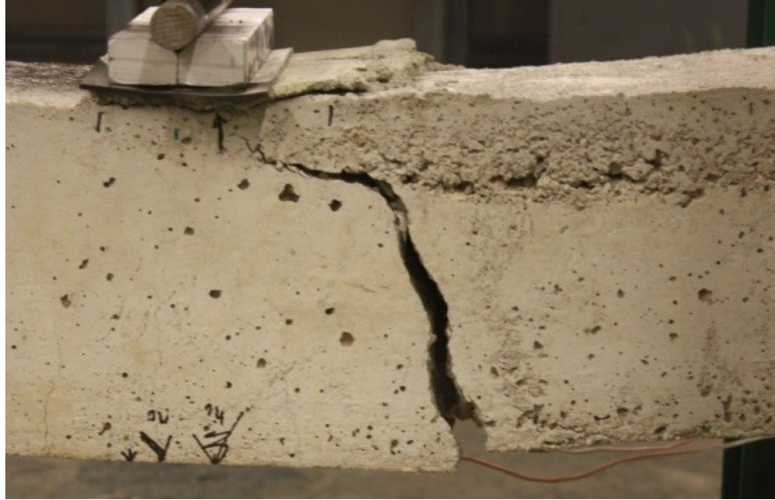
Figure 57: Primary flexural crack in IIIa-2
