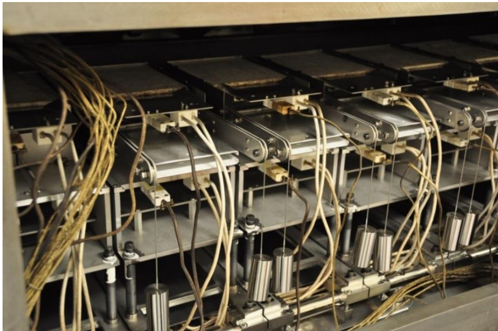
Figure 3-8: ARDS source hardware inside vacuum system
