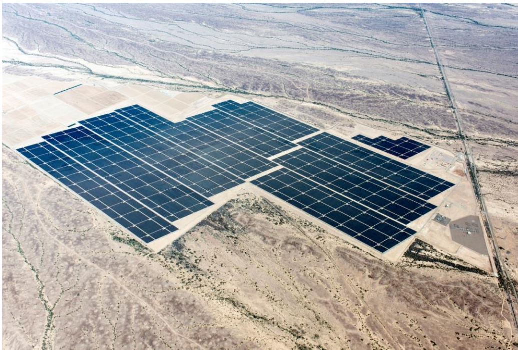
Figure 1-11: Agua Caliente solar farm, First Solar [20]
