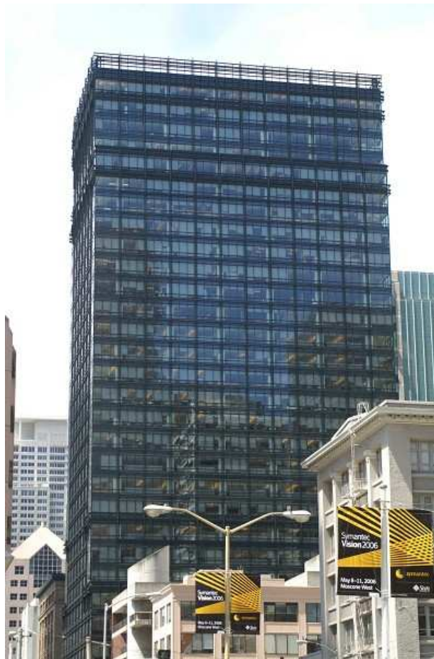
Figure 3-2 JP Morgan-Chase building in San Francisco, CA (Structure)
