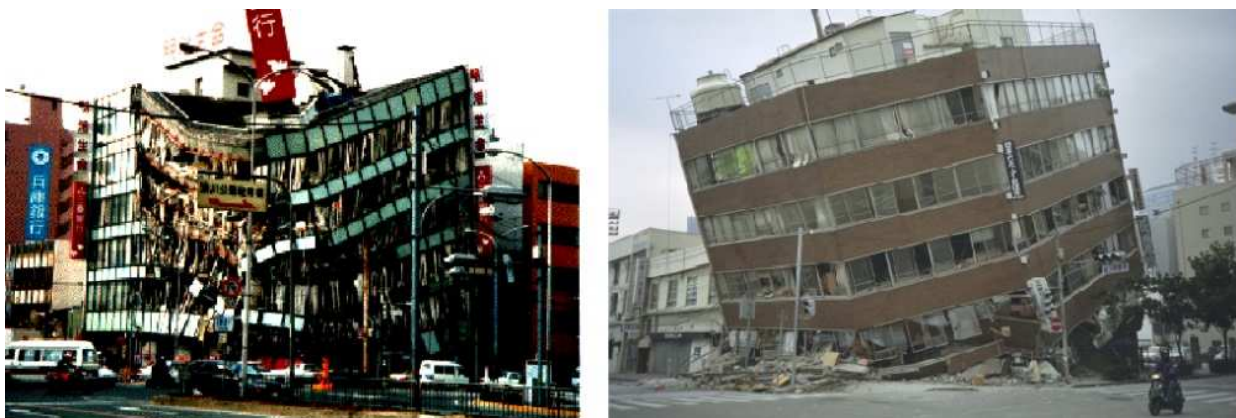
Figure 2-2 Collapsing Structures under Kobe Earthquake
