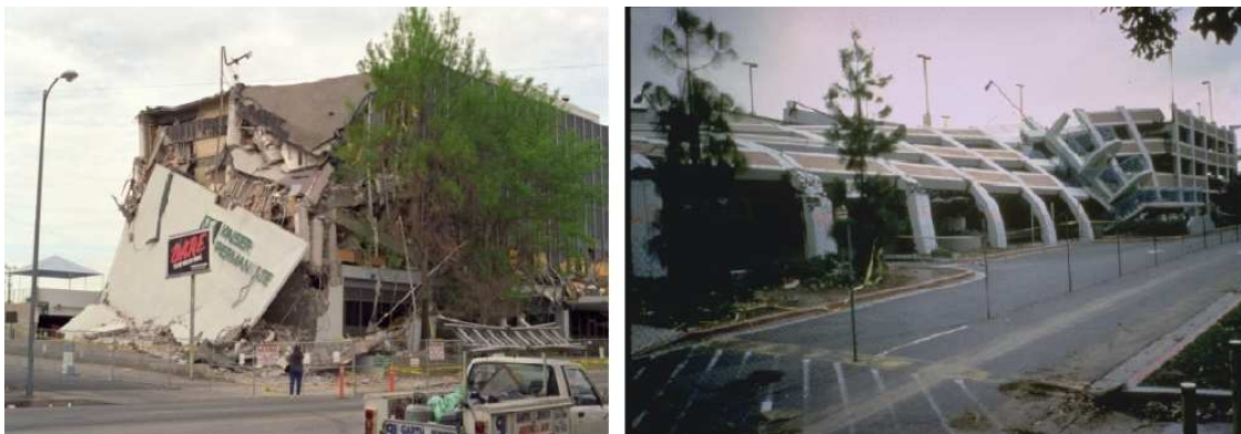
Figure 2-1 Building Collapse Consequences by the Northridge Earthquake
