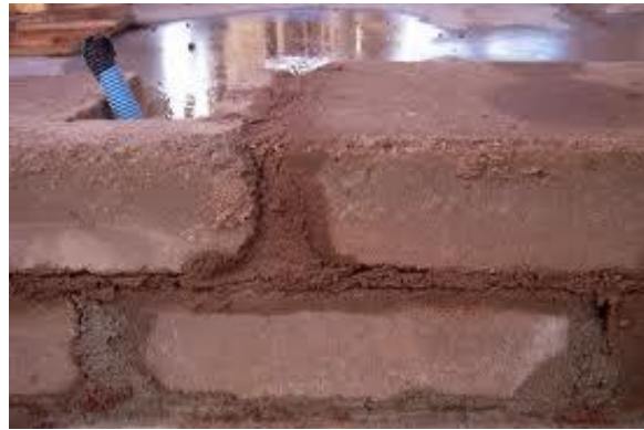
Figure 5: Compressed earth block wall under construction
