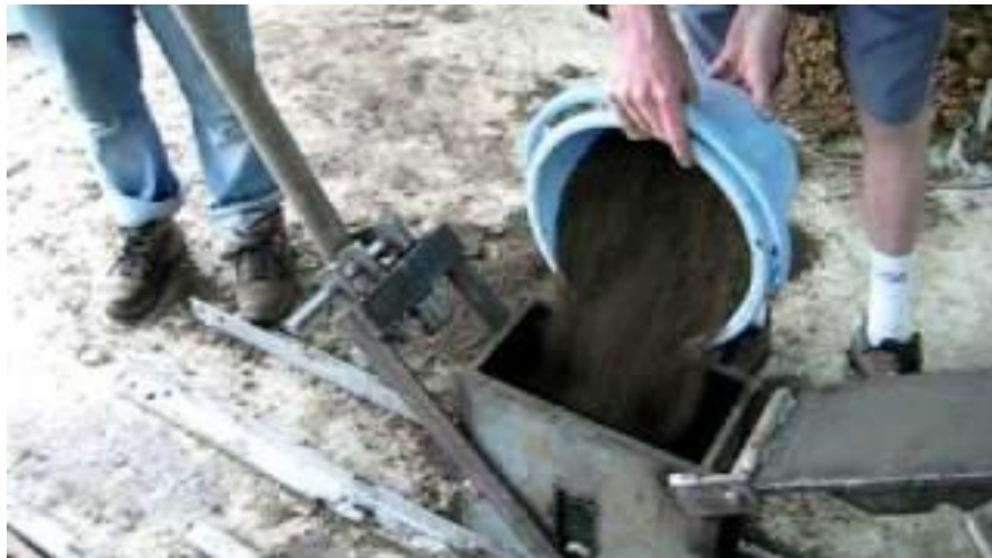
Figure 4: Preparation of typical earth block mix
