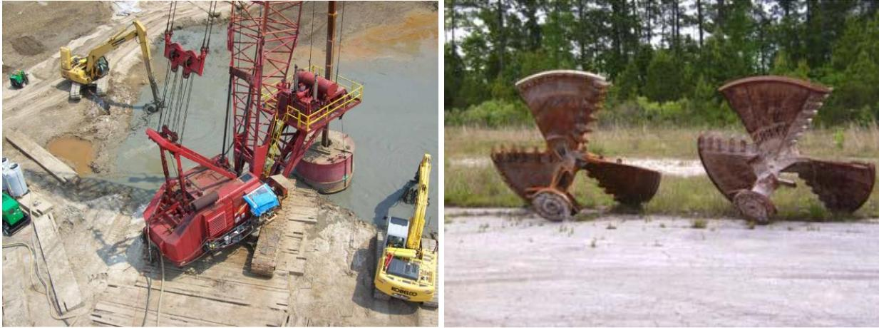
**Figure 2-2. Soil mixing equipment (left) used for ZVI-Clay soil mixing at Camp Lejeune, Site 89, included a crane, crane-mounted rotary table, and hollow kelly bar. Mixing was completed using 3.0-m diameters augers (right).**
