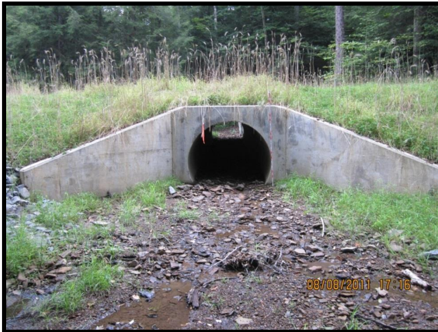
FIGURE 288: LOOKING UPSTREAM AT THE SITE 3 OUTLET
