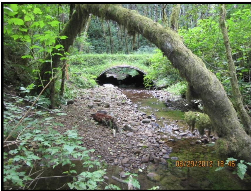
FIGURE 250: LOOKING DOWNSTREAM AT THE INLET TRANSITION ZONE AND STRUCTURE INLET AT NORTH FORK INDIAN
