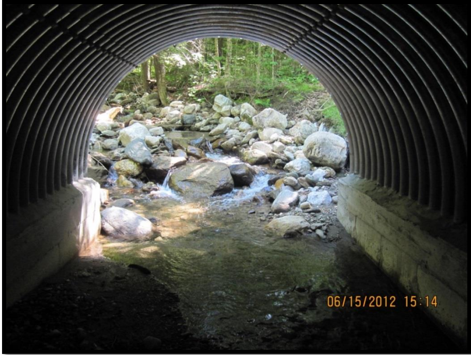
FIGURE 206: LOOKING UPSTREAM AT THE INLET TRANSITION ZONE FROM WITHIN THE JOE SMITH STRUCTURE
