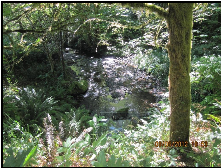
FIGURE 58: LOOKING DOWNSTREAM, FROM THE TOP OF THE STRUCTURE, AT THE BAYS CREEK OUTLET TRANSITION ZONE
