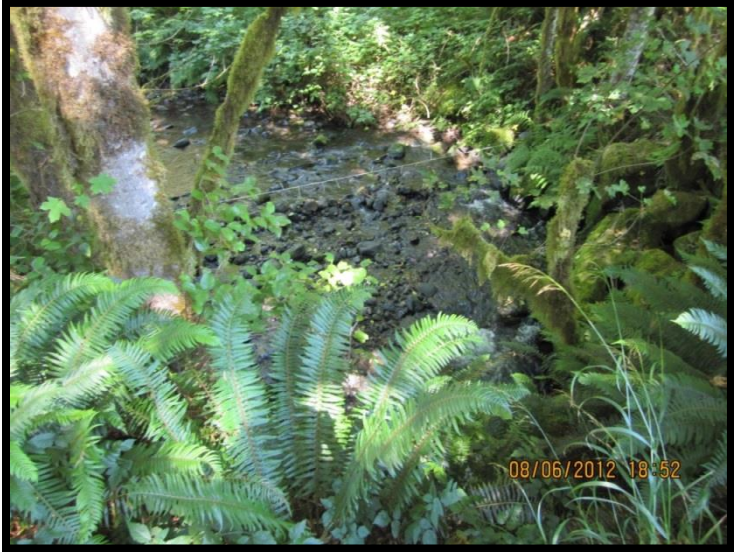
FIGURE 55: LOOKING AT THE BAYS CREEK INLET TRANSITION ZONE FROM THE TOP OF THE STRUCTURE
