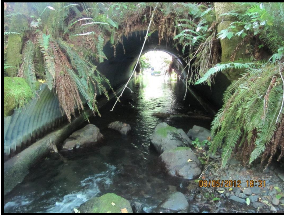
FIGURE 61: LOOKING DOWNSTREAM THROUGH THE BAYS CREEK STRUCTURE
