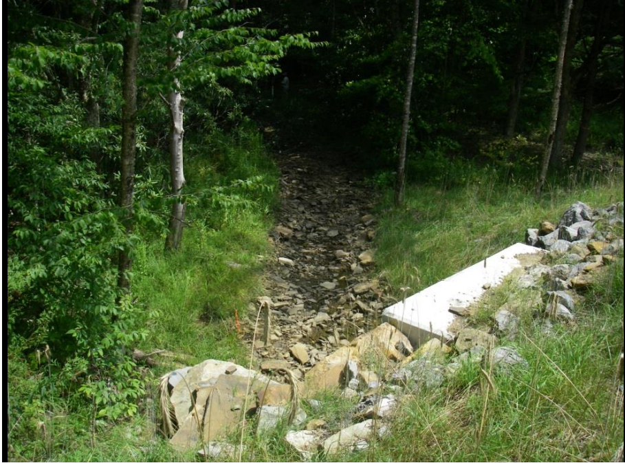
FIGURE 363: LOOKING AT THE INLET TRANSITION ZONE FROM THE TOP OF THE WF01 STRUCTURE
