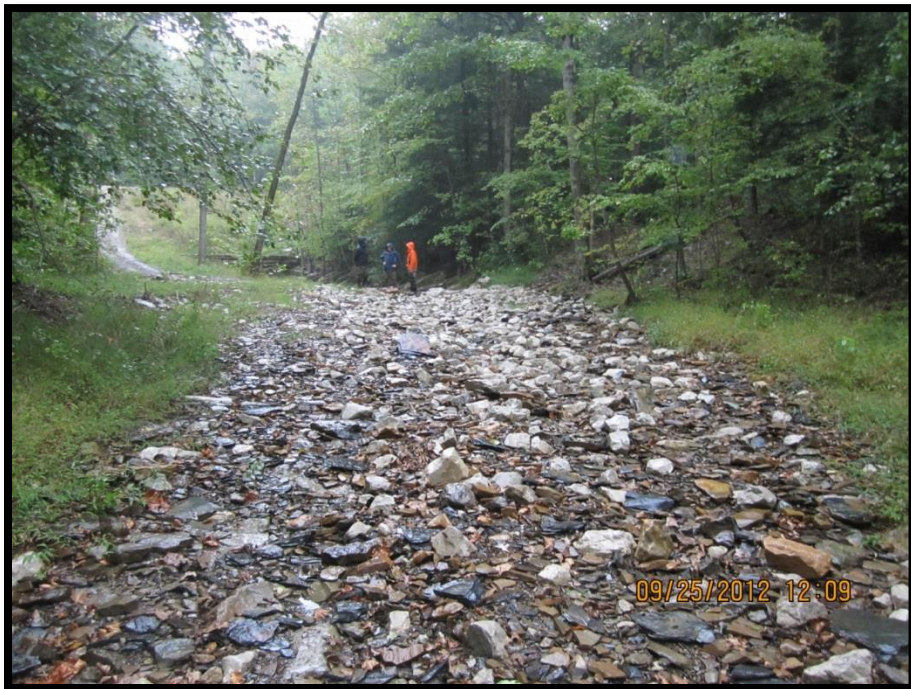
FIGURE 125: THE DRY CONSTRUCTED RIFFLE AT CANEY CREEK
