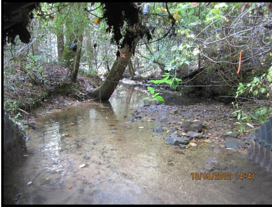
FIGURE 70: WITHIN THE BIG LICK STRUCTURE, LOOKING DOWNSTREAM AT THE OUTLET TRANSITION ZONE
