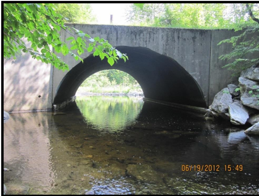
FIGURE 357: UTLEY BROOK STRUCTURE INLET WITH BOULDER RIP-RAP
