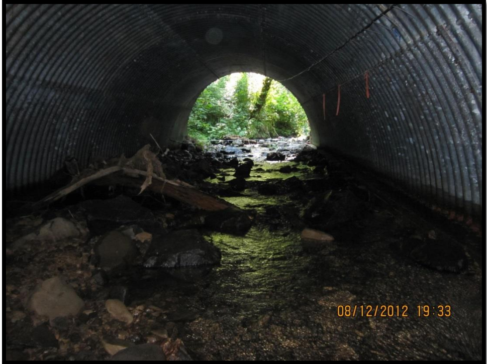
FIGURE 22: LOOKING UPSTREAM WITHIN THE LOWER STILLWELL STRUCTURE
