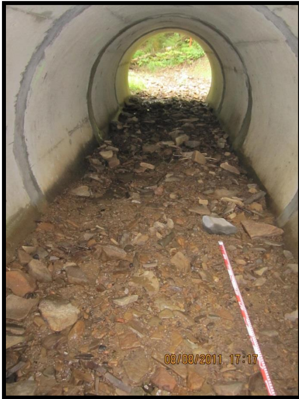
FIGURE 290: LOOKING UPSTREAM WITHIN THE SITE 3 STRUCTURE
