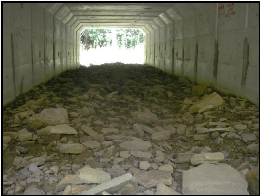
FIGURE 368: LOOKING UPSTREAM WITHIN THE WF01 STRUCTURE
