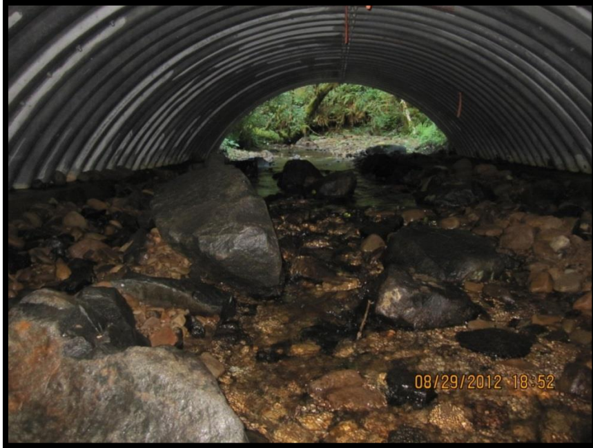
FIGURE 253: LOOKING UPSTREAM WITHIN THE NORTH FORK INDIAN STRUCTURE; SSR2 AND SR1 CHANNEL UNITS VISIBLE
