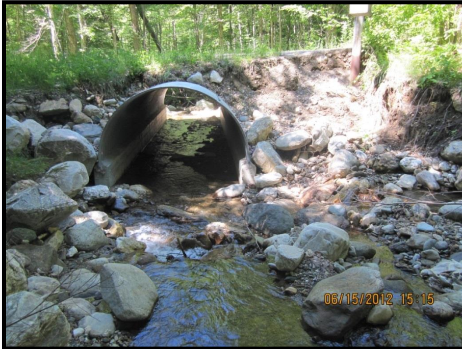
FIGURE 203: LOOKING DOWNSTREAM AT THE JOE SMITH STRUCTURE INLET
