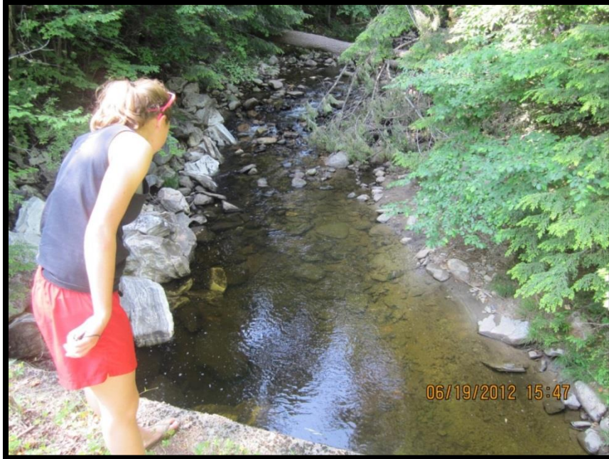
FIGURE 356: LOOKING UPSTREAM AT THE INLET TRANSITION ZONE AND NATURAL CHANNEL FROM THE TOP OF THE UTLEY BROOK STRUCTURE
