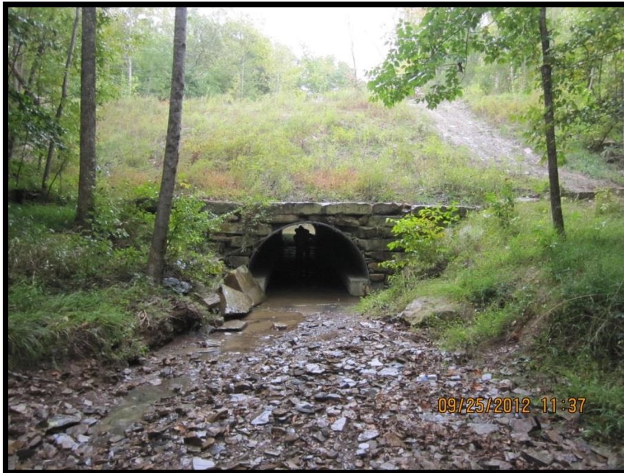
FIGURE 121: LOOKING DOWNSTREAM AT THE CANEY CREEK STRUCTURE INLET
