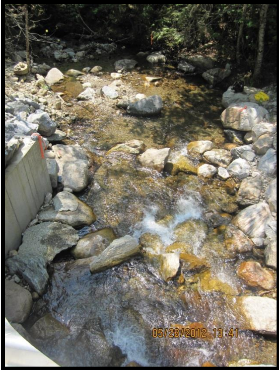
FIGURE 314: LOOKING DOWNSTREAM AT THE SPARKS BROOK OUTLET TRANSITION ZONE (FROM THE TOP OF THE STRUCTURE)
