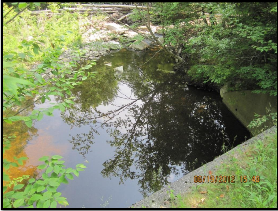
FIGURE 358: VIEW OF THE OUTLET TRANSITION ZONE FROM THE TOP OF THE UTLEY BROOK STRUCTURE
