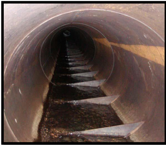
FIGURE 4: HYDRAULIC DESIGN EXAMPLE STRUCTURE RETROFIT
