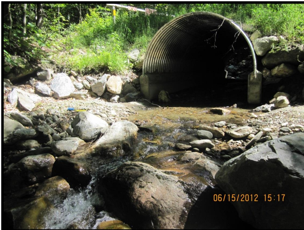
FIGURE 205: LOOKING UPSTREAM AT THE JOE SMITH STRUCTURE OUTLET
