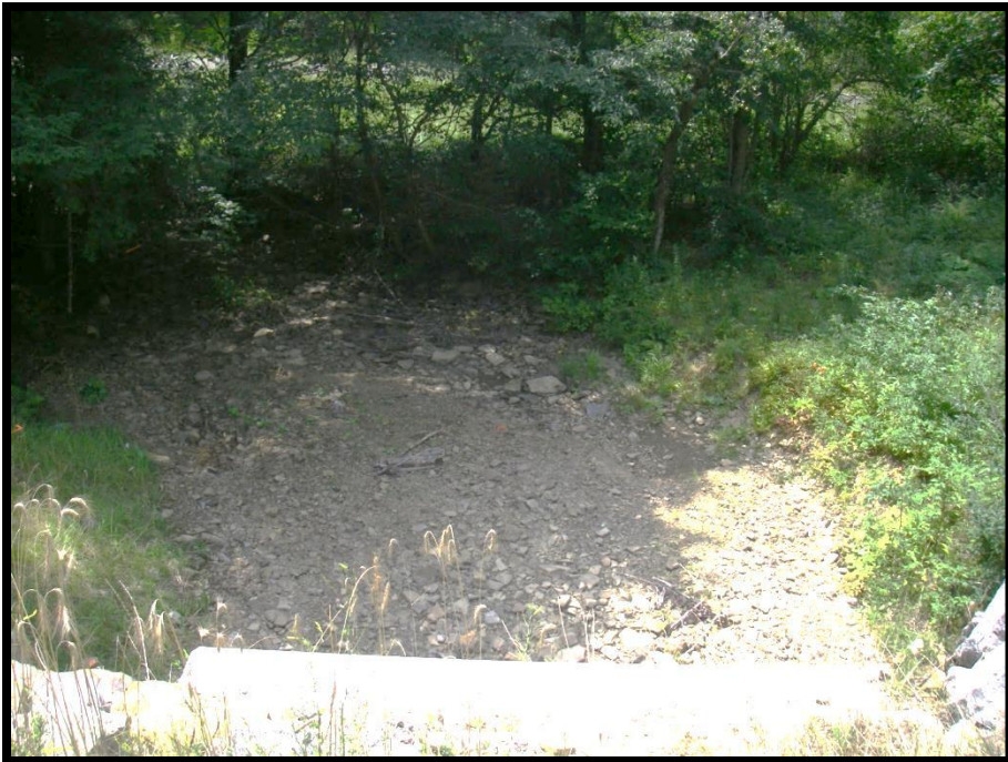
FIGURE 366: LOOKING AT THE WF01 OUTLET TRANSITION ZONE FROM THE TOP OF THE STRUCTURE
