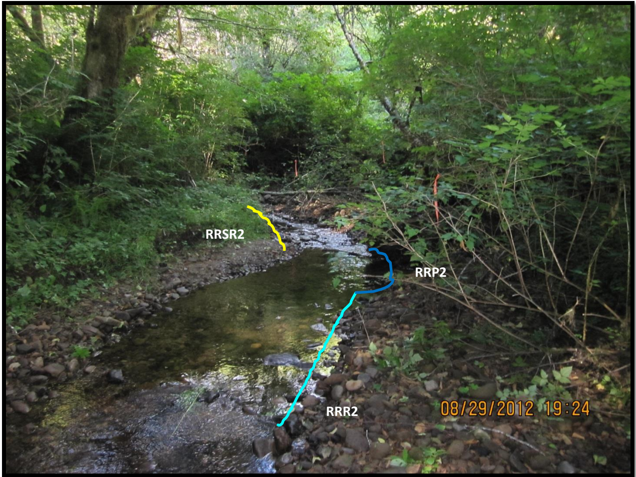
FIGURE 255: LOOKING AT THE NORTH FORK INDIAN REPRESENTATIVE REACH FOR THE STEEPER DESIGN SLOPE SECTION; RRSR2, RRP2, AND RRR2 UNITS ARE VISIBLE
