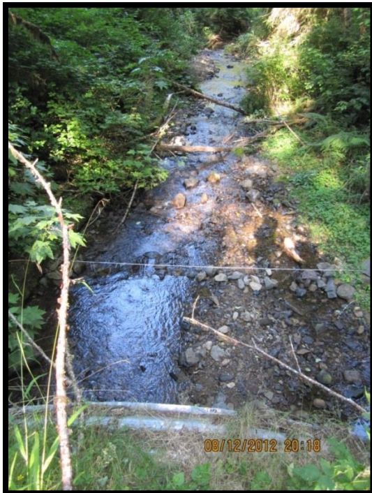
FIGURE 217: LOOKING DOWNSTREAM AT THE LOWER STILLWELL OUTLET TRANSITION ZONE FROM THE TOP OF THE STRUCTURE
