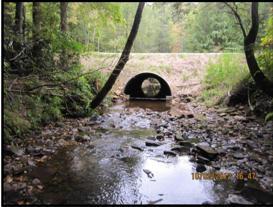
FIGURE 129: LOOKING DOWNSTREAM AT THE DOG SLAUGHTER STRUCTURE INLET TRANSITION ZONE AND INLET
