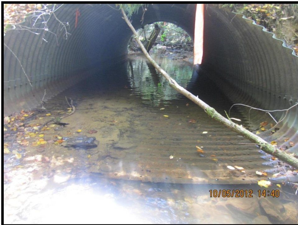
FIGURE 69: LOOKING DOWNSTREAM WITHIN THE BIG LICK STRUCTURE
