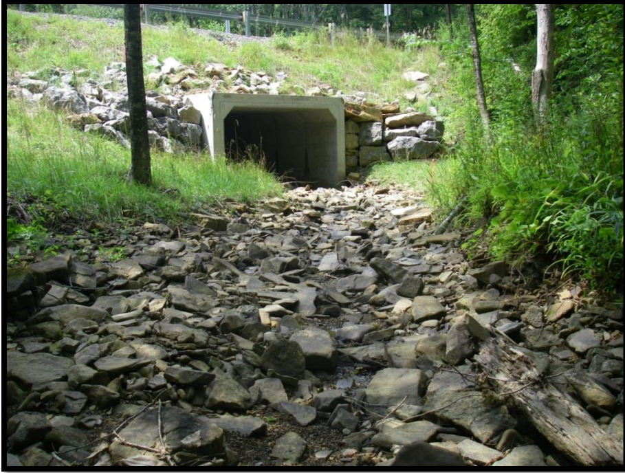
FIGURE 365: LOOKING DOWNSTREAM AT THE WF01 INLET TRANSITION ZONE AND STRUCTURE INLET
