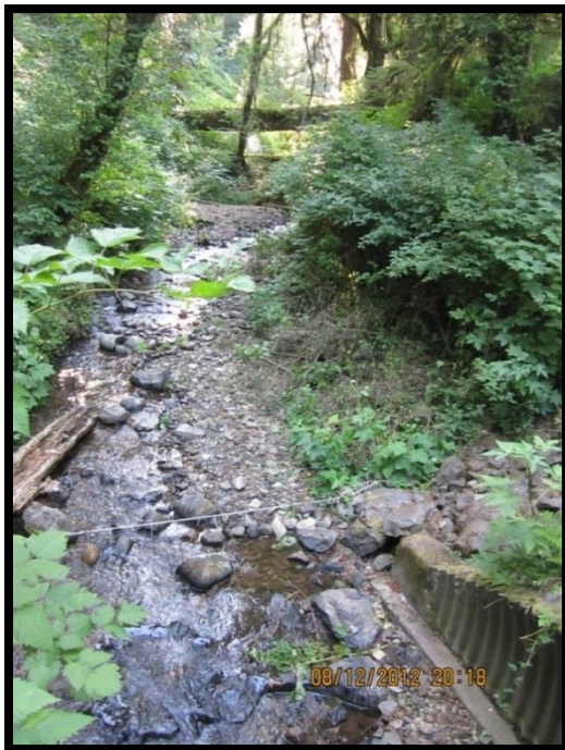
FIGURE 215: LOOKING UPSTREAM AT THE INLET TRANSITION ZONE FROM THE TOP OF THE LOWER STILLWELL STRUCTURE
