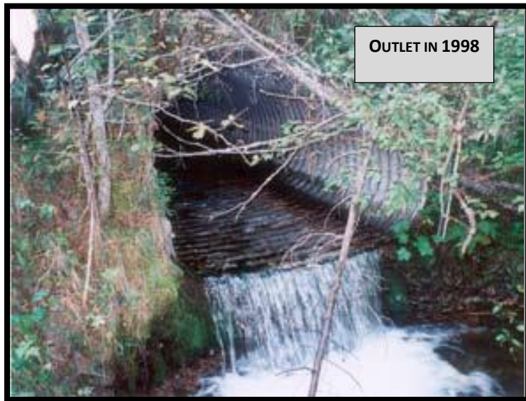
FIGURE 3: UNDERSIZED CULVERT OUTLET OVER TIME
