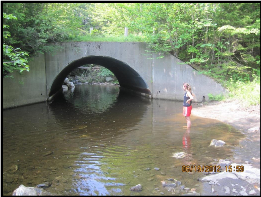
FIGURE 359: LOOKING UPSTREAM AT THE UTLEY BROOK STRUCTURE OUTLET
