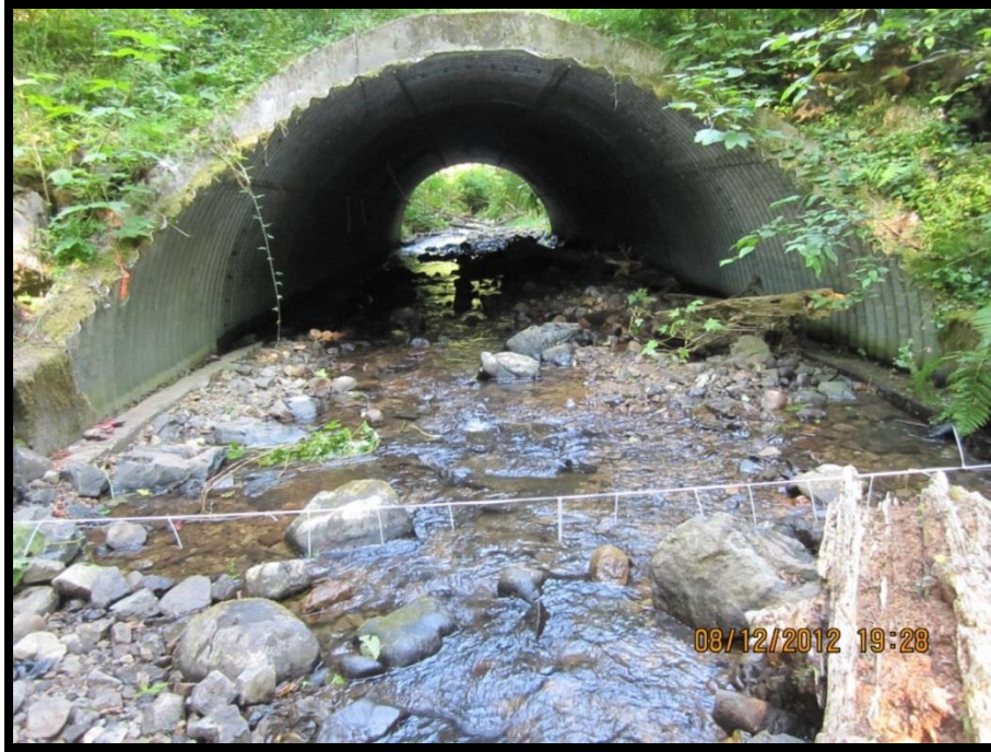
FIGURE 214: LOOKING DOWNSTREAM AT THE STRUCTURE INLET AT LOWER STILLWELL
