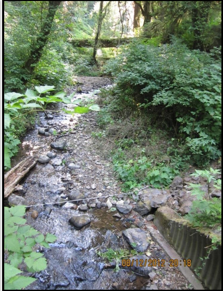
FIGURE 24: LOOKING UPSTREAM AT THE INLET TRANSITION ZONE FROM THE TOP OF THE CULVERT AT LOWER STILLWELL
