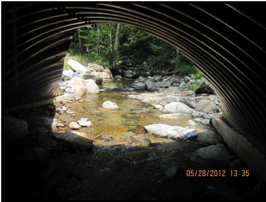
FIGURE 313: LOOKING UPSTREAM AT THE SPARKS BROOK INLET TRANSITION ZONE
