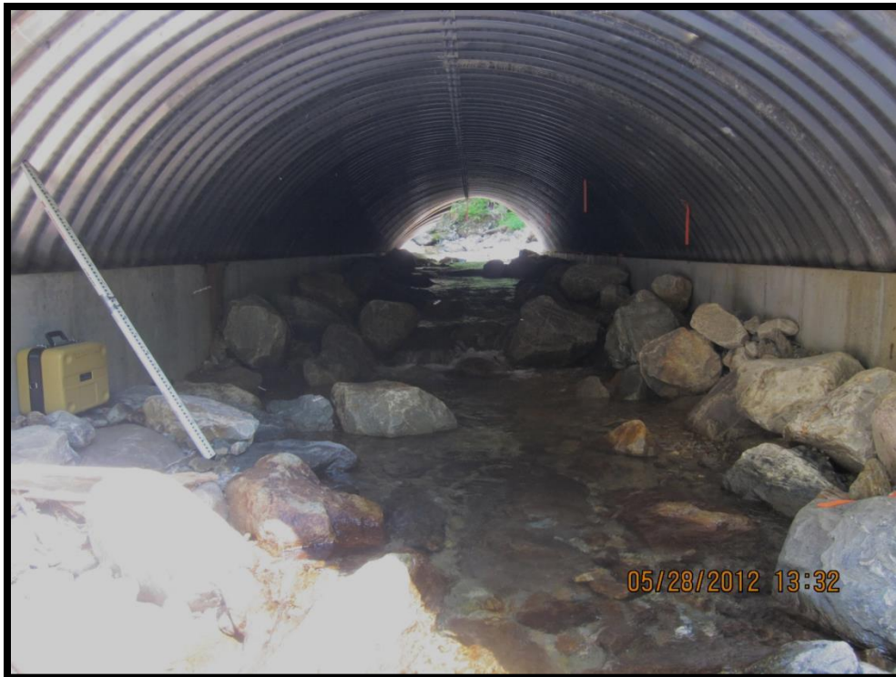
FIGURE 317: LOOKING UPSTREAM FROM WITHIN THE SPARKS BROOK STRUCTURE
