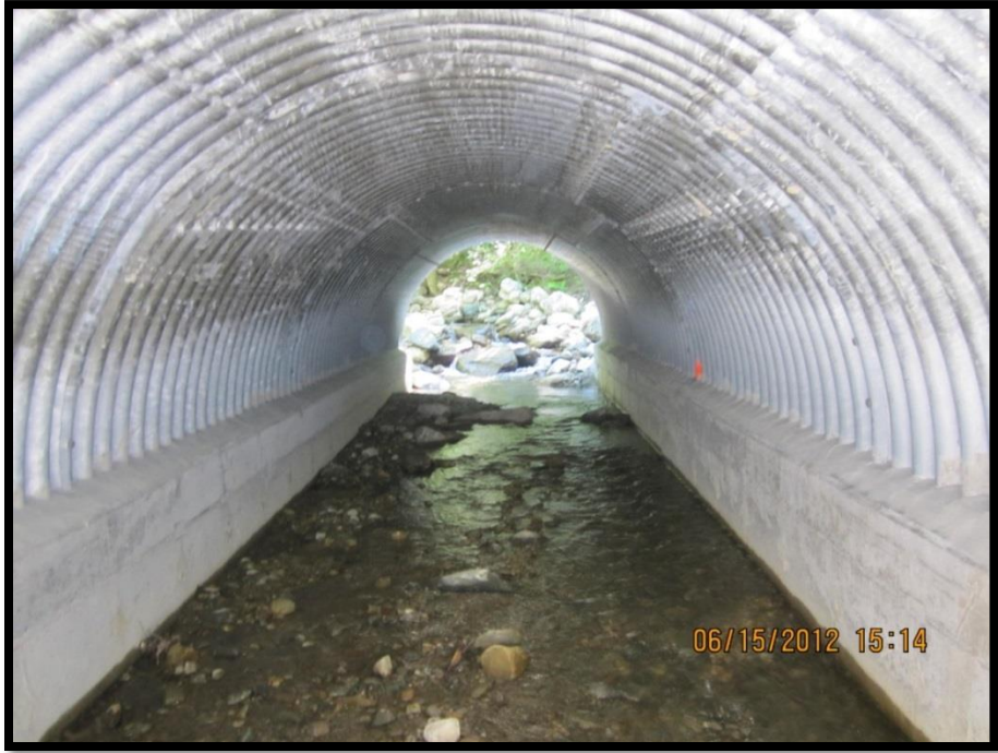
FIGURE 207: LOOKING DOWNSTREAM WITHIN THE JOE SMITH STRUCTURE
