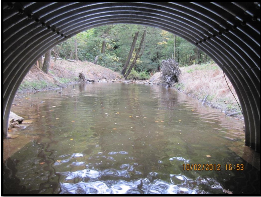
FIGURE 131: LOOKING DOWNSTREAM THROUGH THE DOG SLAUGHTER STRUCTURE OUTLET
