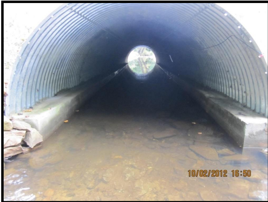
FIGURE 130: LOOKING DOWNSTREAM FROM THE DOG SLAUGHTER STRUCTURE INLET
