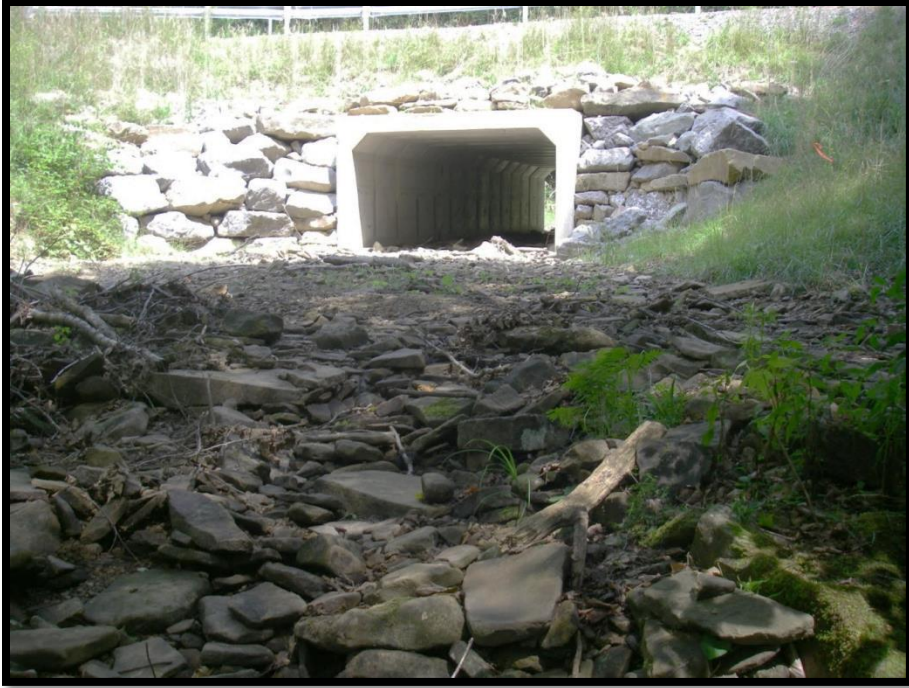
FIGURE 367: LOOKING UPSTREAM AT THE WF01 OUTLET TRANSITION ZONE AND STRUCTURE
