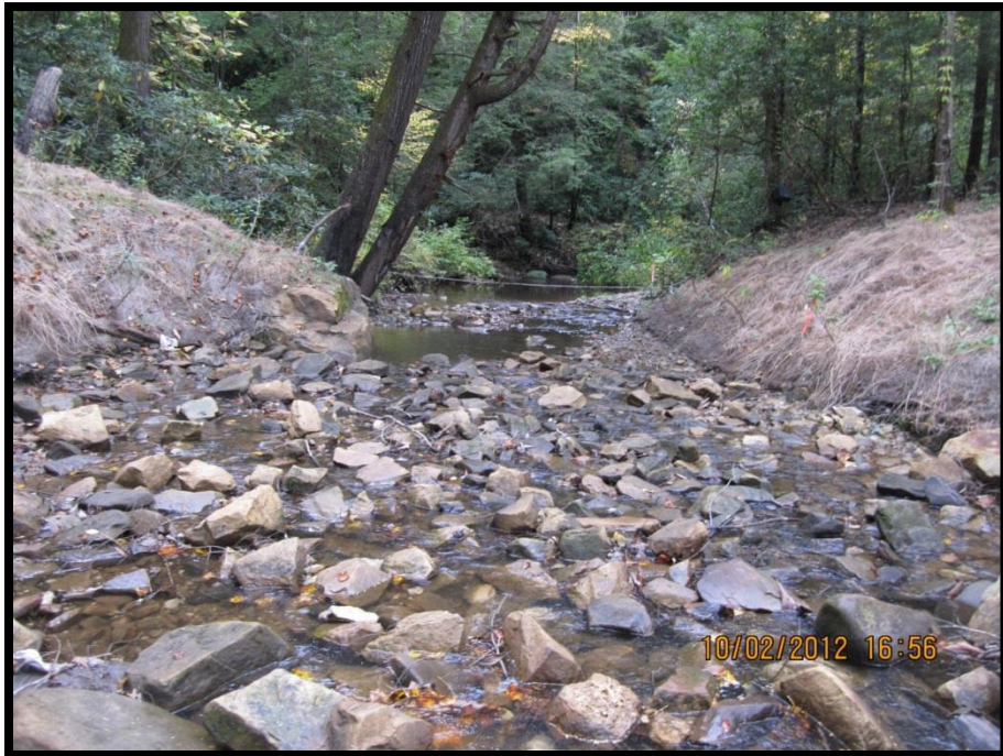
FIGURE 132: WITHIN THE CONSTRUCTED RIFFLE WHICH BACKWATERS THE DOG SLAUGHTER STRUCTURE; DOWNSTREAM OF THE OUTLET TRANSITION ZONE
