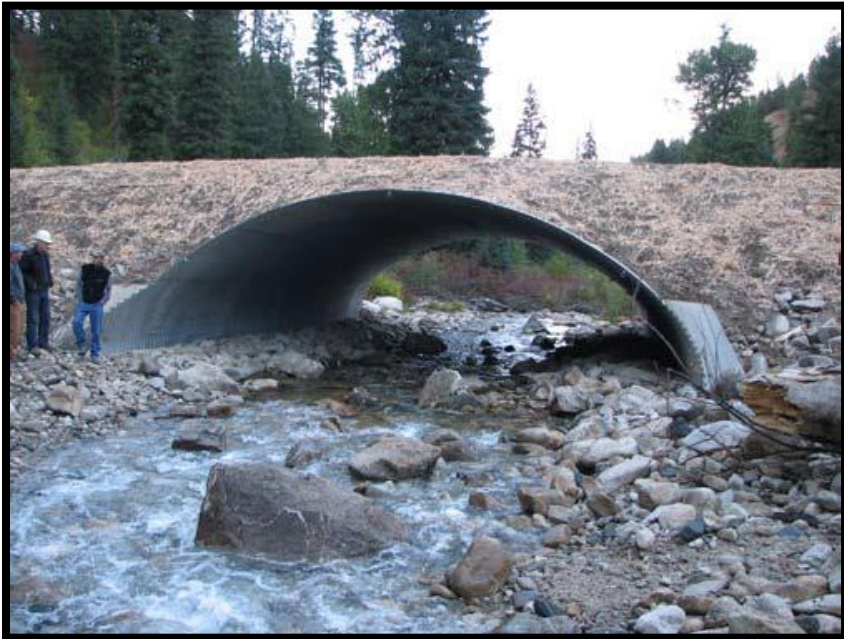
FIGURE 8: ROAD-STREAM CROSSING ON THE BOISE NF, STREAM SIMULATION DESIGN CULVERT POST-REPLACEMENT
