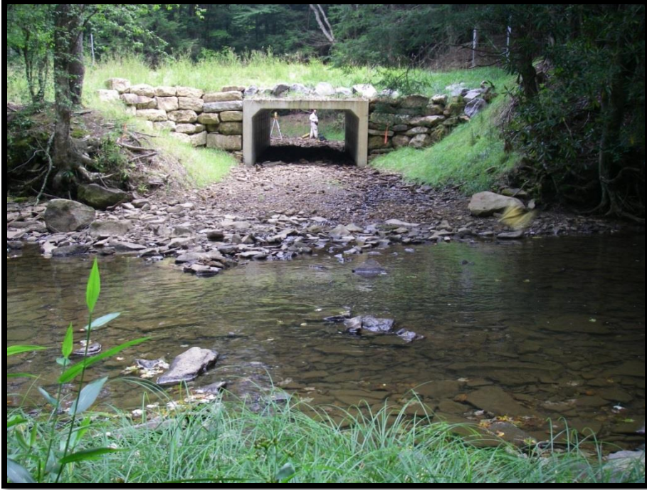
FIGURE 394: LOOKING UPSTREAM AT THE WF02 OUTLET AND THE CONFLUENCE OF COVE RUN AND THE GREENBRIER RIVER
