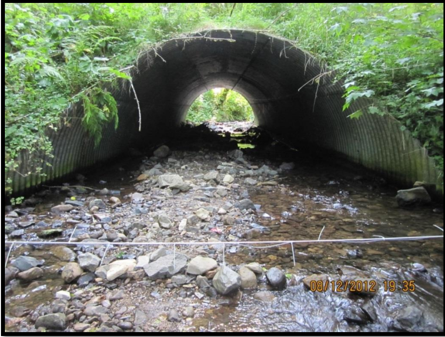
FIGURE 218: LOOKING UPSTREAM AT THE LOWER STILLWELL OUTLET
