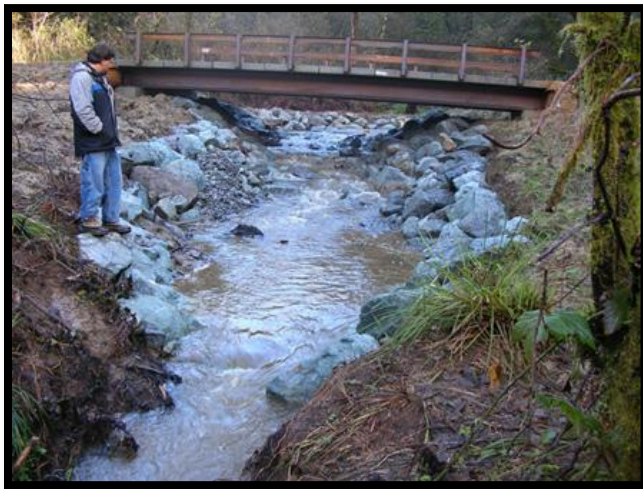
FIGURE 6: A ROAD-STREAM CROSSING ROUGHENED CHANNEL DESIGN
