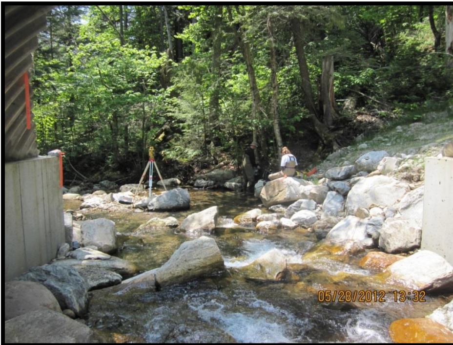
FIGURE 315: LOOKING DOWNSTREAM AT THE SPARKS BROOK OUTLET TRANSITION ZONE (FROM WITHIN THE STRUCTURE)
