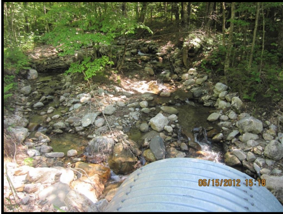
FIGURE 202: LOOKING AT THE JOE SMITH INLET TRANSITION ZONE FROM THE TOP OF THE STRUCTURE
