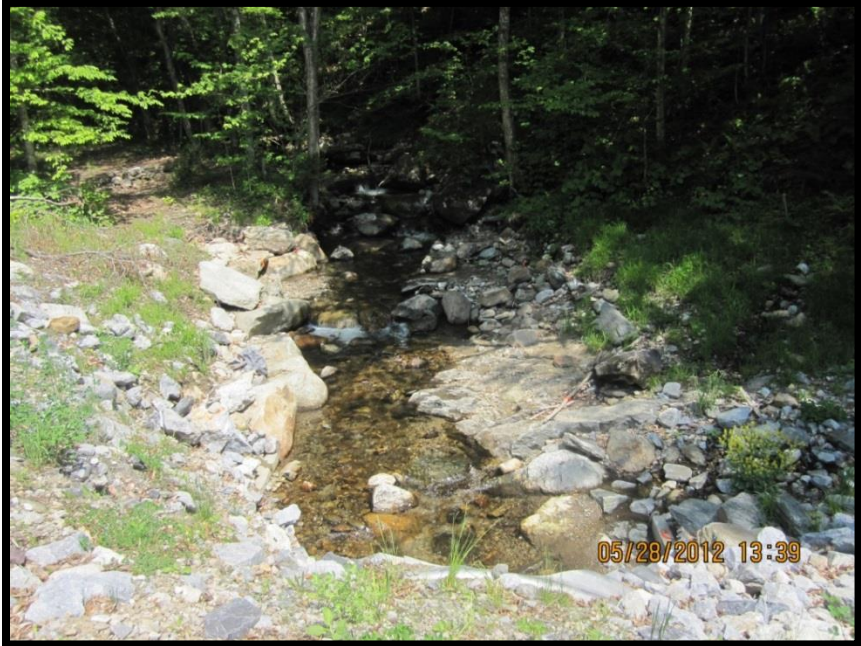
FIGURE 310: LOOKING UPSTREAM AT THE INLET TRANSITION ZONE FROM THE TOP OF THE SPARKS BROOK STRUCTURE
