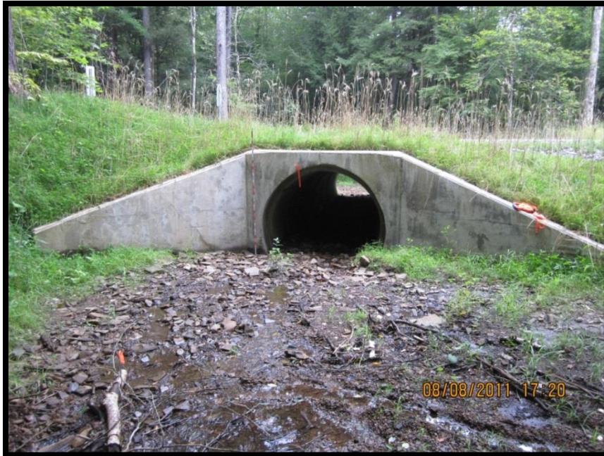
FIGURE 287: LOOKING DOWNSTREAM AT THE SITE 3 INLET
