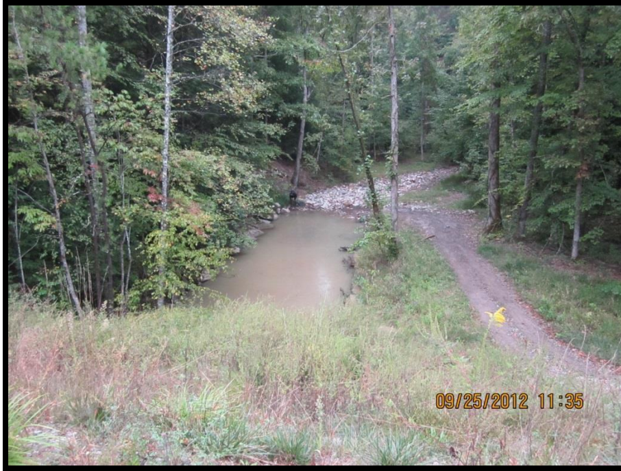
FIGURE 122: LOOKING DOWNSTREAM AT THE OUTLET TRANSITION ZONE AND CONSTRUCTED RIFFLE FROM THE TOP OF THE CANEY CREEK STRUCTURE
