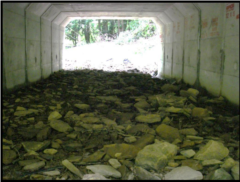
FIGURE 395: LOOKING UPSTREAM WITHIN THE WF02 STRUCTURE
