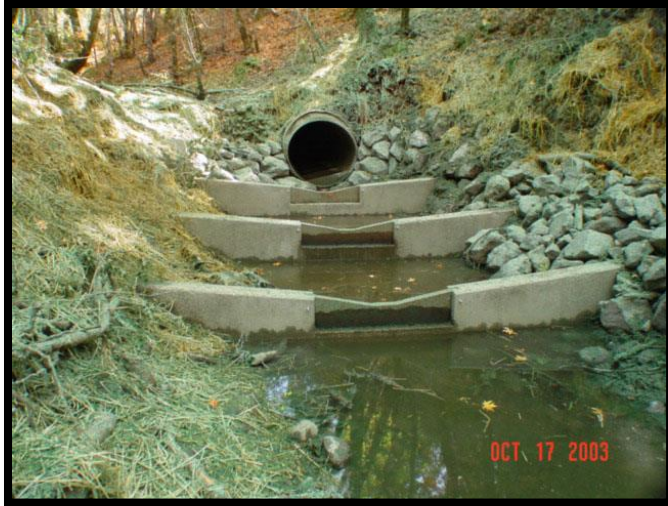
FIGURE 5: HYDRAULIC DESIGN EXAMPLE OUTLET
