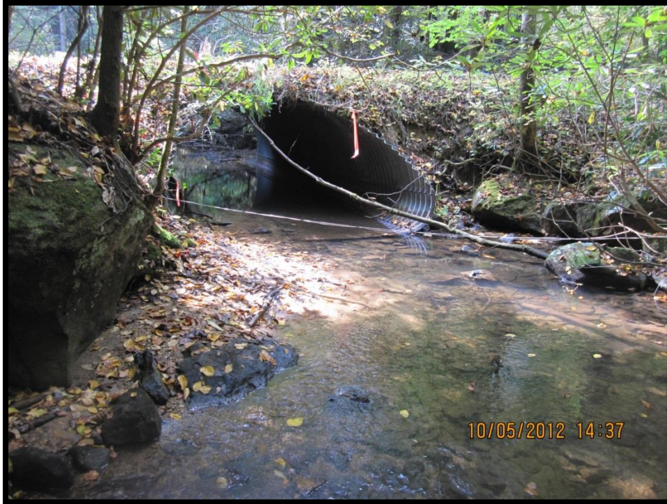
FIGURE 68: LOOKING DOWNSTREAM AT THE BIG LICK STRUCTURE INLET
