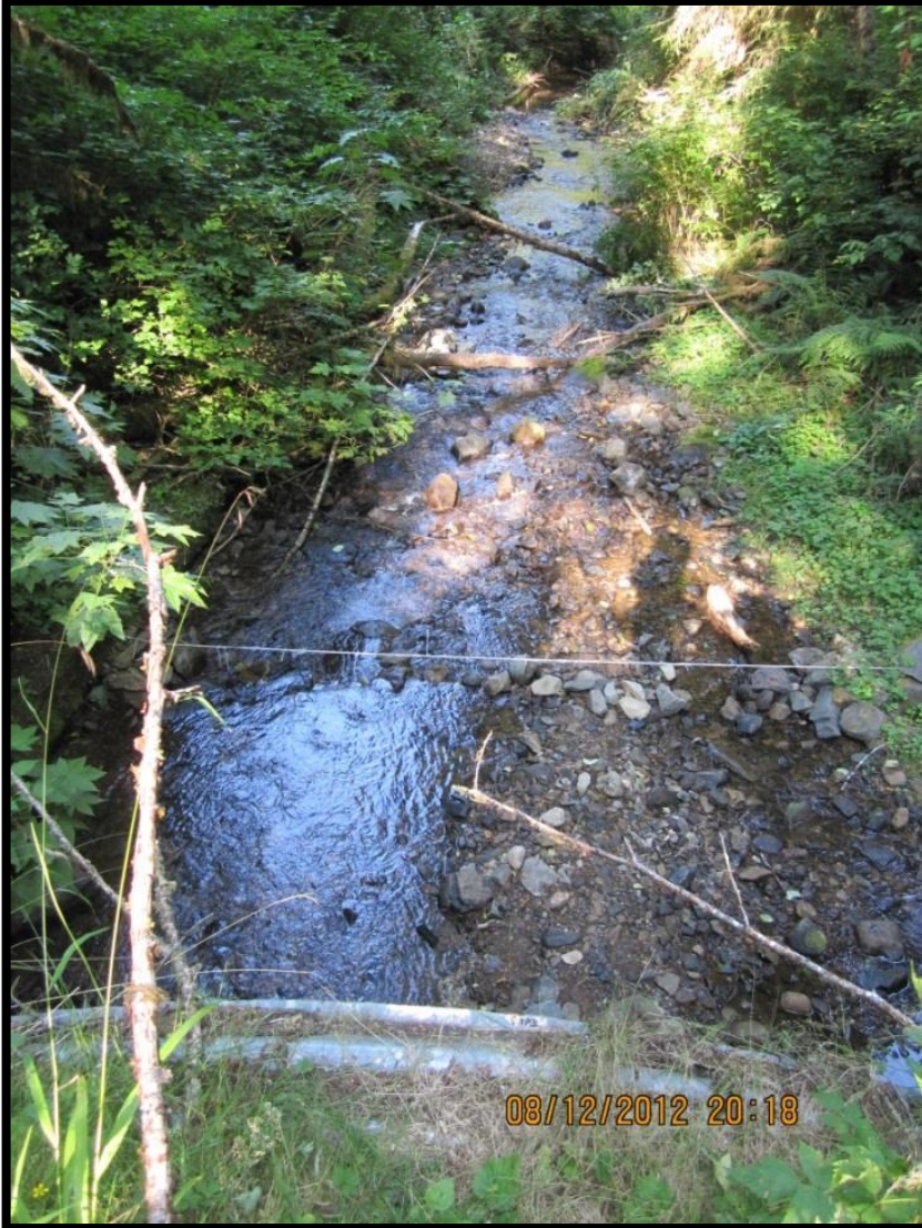
FIGURE 25: LOOKING DOWN-STREAM AT THE OUTLET TRANSITION ZONE FROM THE TOP OF THE CULVERT AT LOWER STILLWELL
