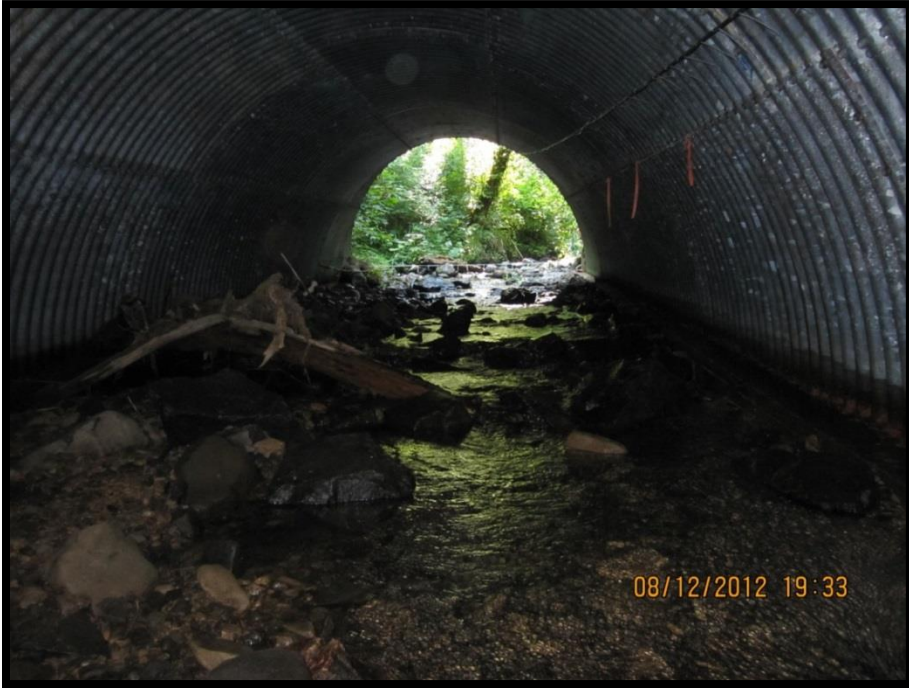
FIGURE 219: LOOKING UPSTREAM WITHIN THE LOWER STILLWELL STRUCTURE
