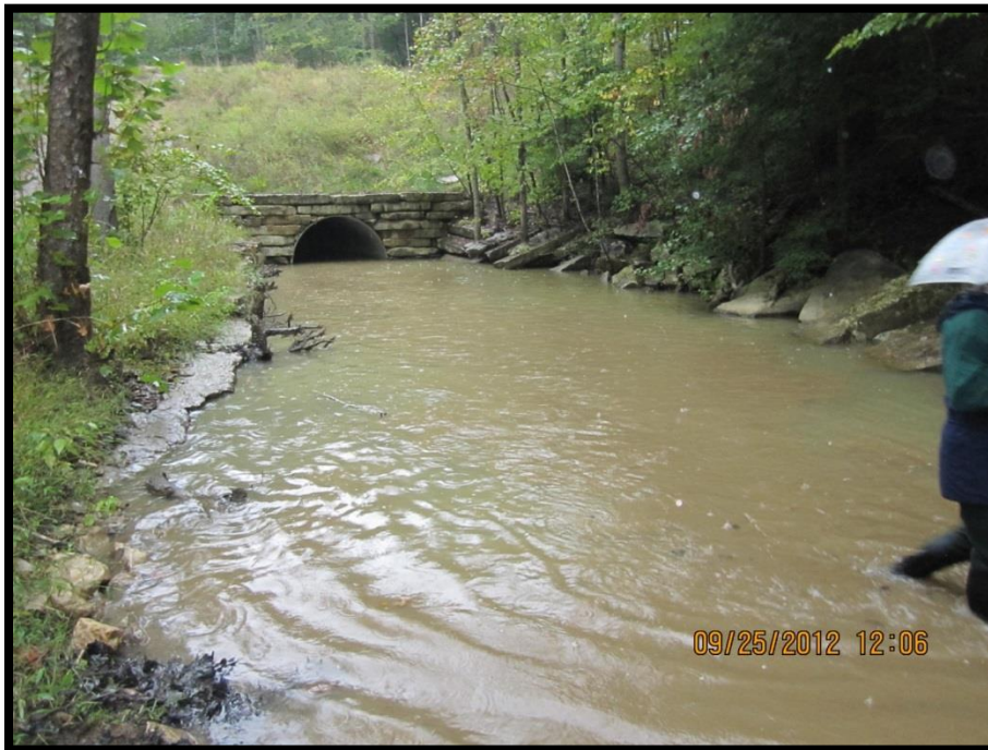
FIGURE 123: LOOKING UPSTREAM AT THE CANEY CREEK STRUCTURE OUTLET AND POOL WITHIN THE OUTLET TRANSITION ZONE
