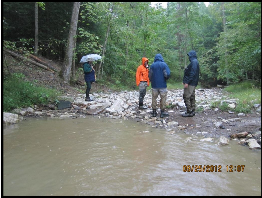
FIGURE 124: PEOPLE STANDING ON THE CONSTRUCTED RIFFLE CREST WHICH BACKWATERS THE CANEY CREEK DESIGN POOL
