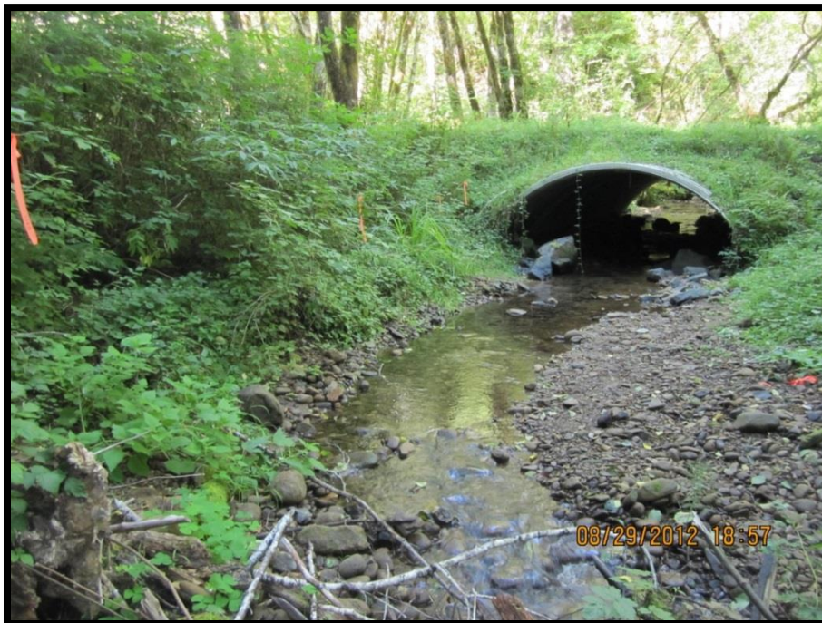
FIGURE 252: LOOKING UPSTREAM AT THE OUTLET TRANSITION ZONE FOR NORTH FORK INDIAN
