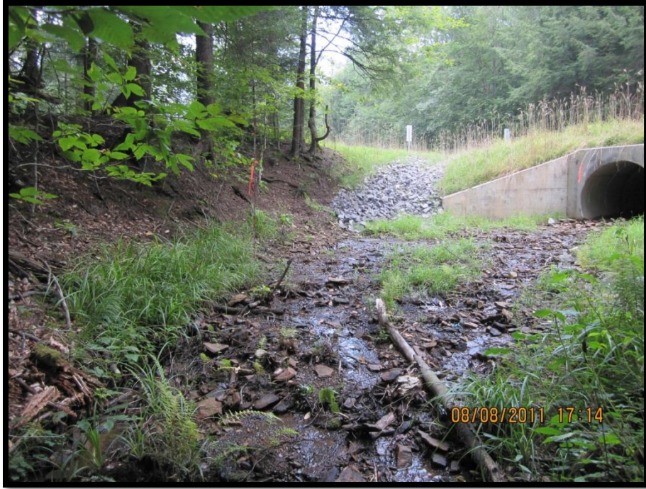
FIGURE 289: LOOKING UPSTREAM AT THE SITE 3 OUTLET TRANSITION ZONE BOUNDARY (MAJOR BREAK IN GRADIENT)
