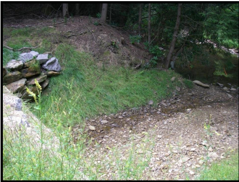
FIGURE 393: LOOKING AT THE OUTLET TRANSITION ZONE AND THE COVE RUN/GREENBRIER CONFLUENCE FROM THE TOP OF THE WF02 STRUCTURE
