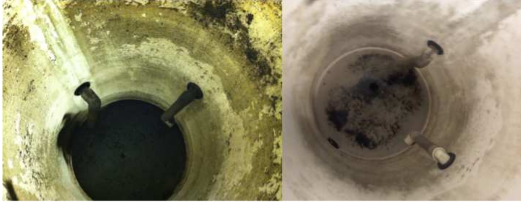
Figure 4.6 Storage Tank Before (left) and After (right) Cleaning
