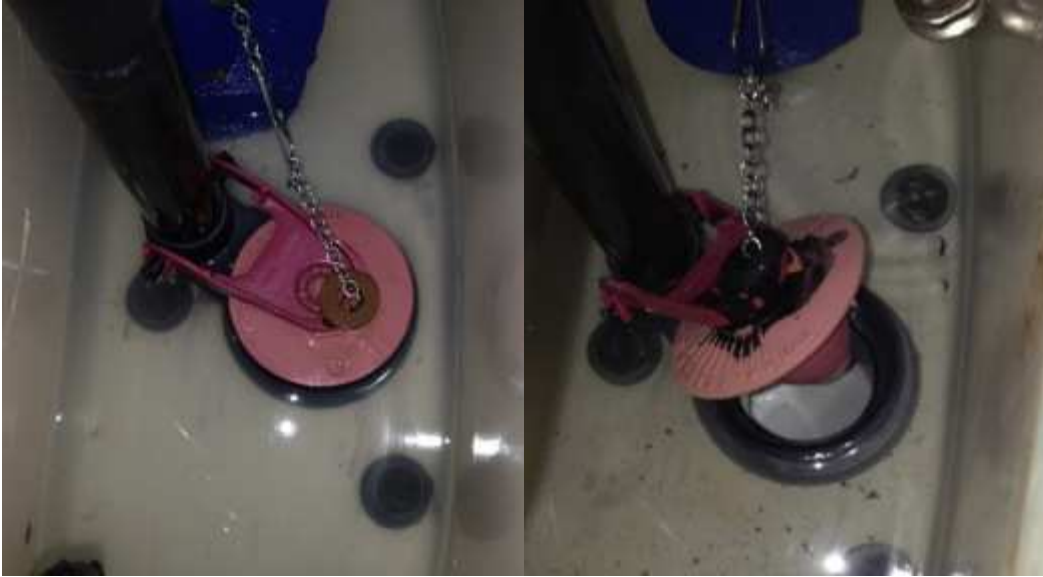
Figure 4.7 Toilet Flapper Monitoring; March 3, 2013 (left), approximately 5 months after operation started. Toilet flapper on May 16, 2013 (right).
