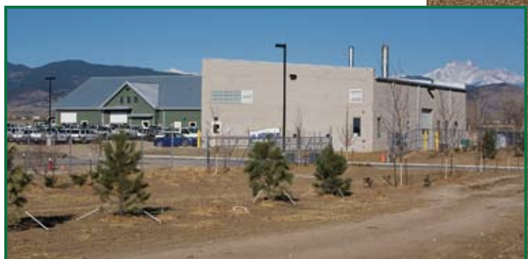
Wood chips from forest treatments heat the new Boulder County Open Space facilities in Longmont. The plant is designed to heat 120,000 square feet.
