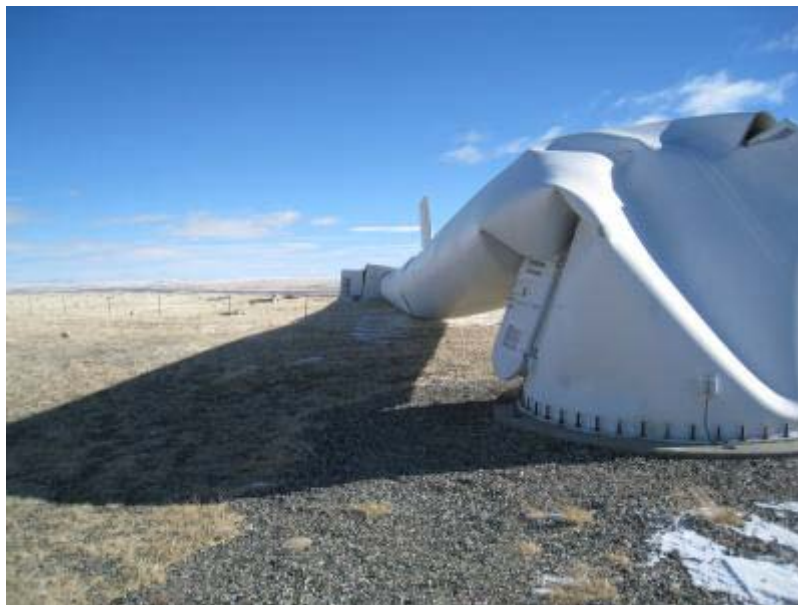
Figure 1-2: Collapse of Wind Turbine Near Arlington, Wyoming (Brome, 2010)
