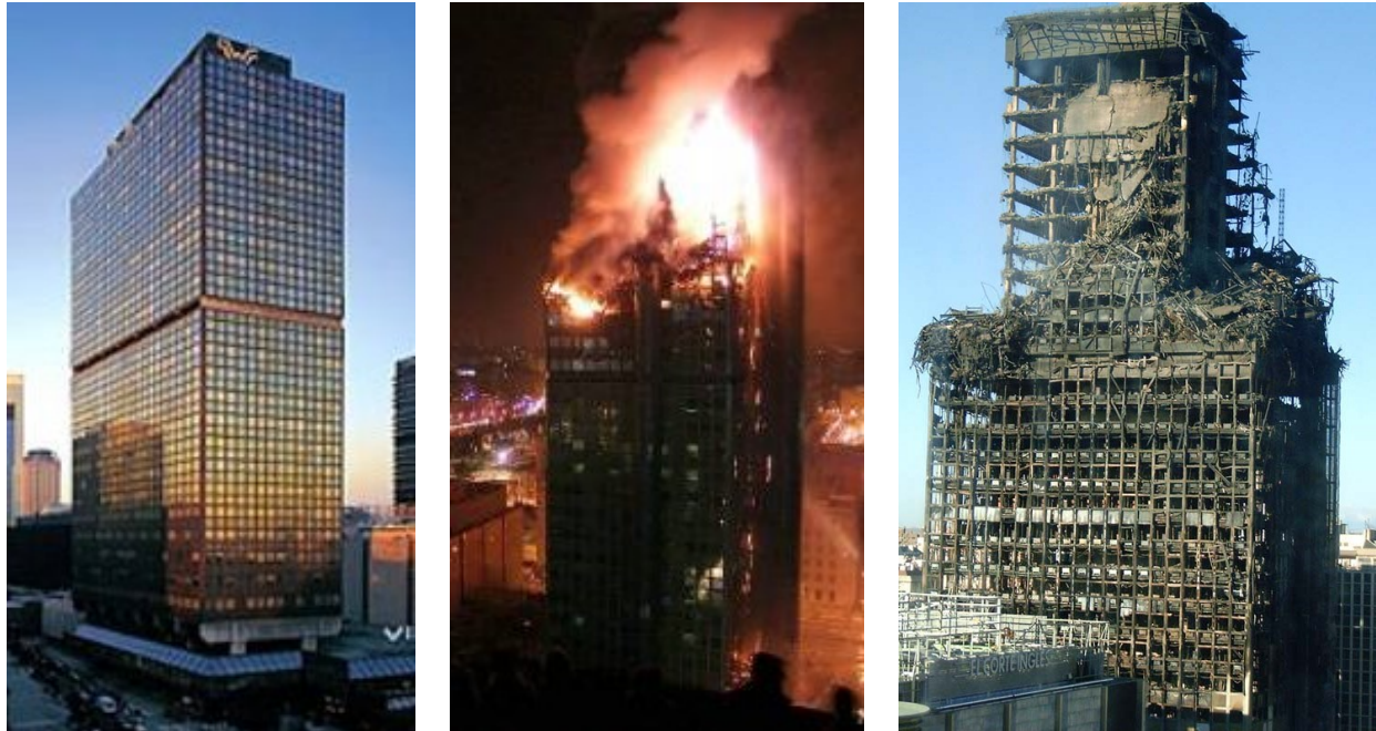
Figure 2-8. Before, During and After Pictures of the 2005 Windsor Building Fire (Meyer, 2012)
