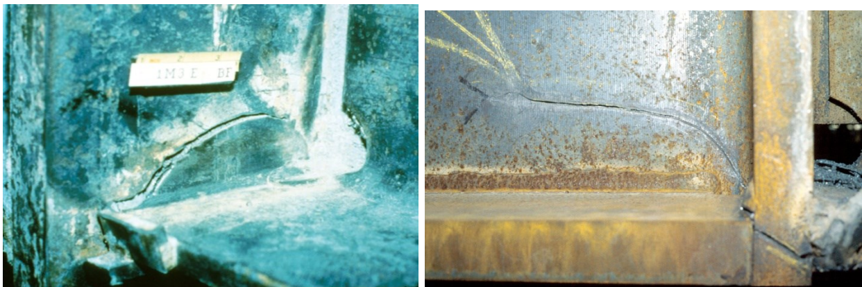
Figure 2-1. Failures Observed in Steel Moment Connections during the Northridge Earthquake (Engelhardt, 2000)
