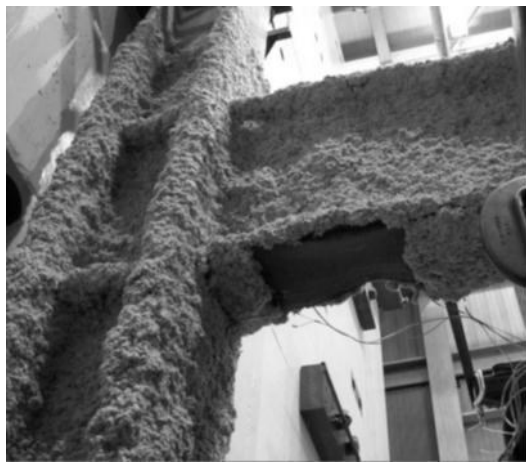
Figure 3-3a. Damaged SFRM insulation at beam hinge region after cyclic loading (Keller and Pessiki, 2012)
